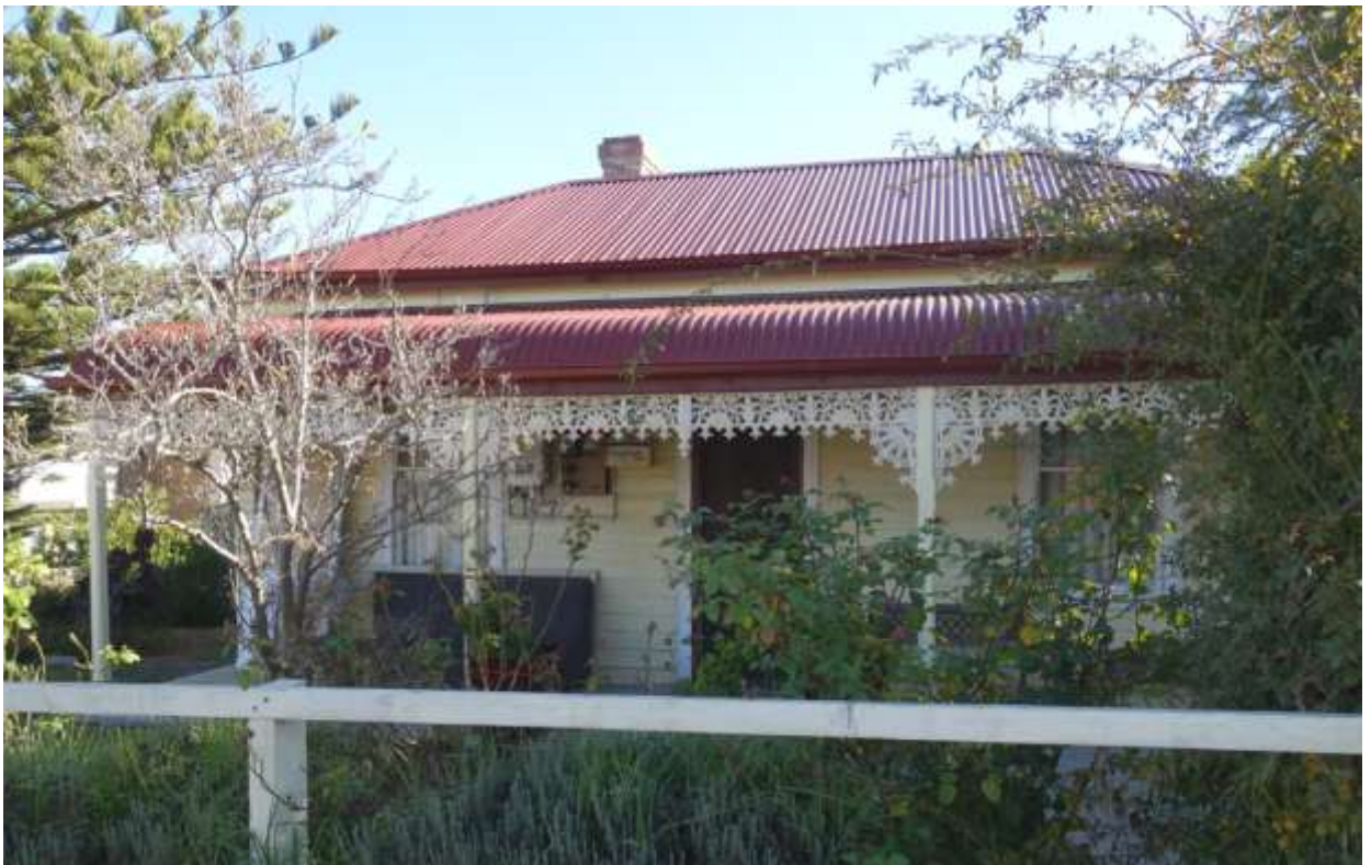
8.24: Former Congregational Manse, 23 Scallan Street. (Source: Landmark Heritage PL, 2024)
