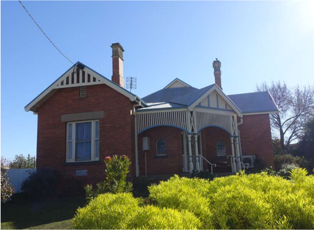
8.21: Former Presbyterian Manse, 9 Scallan Street. (Source: Landmark Heritage PL, 2024)
