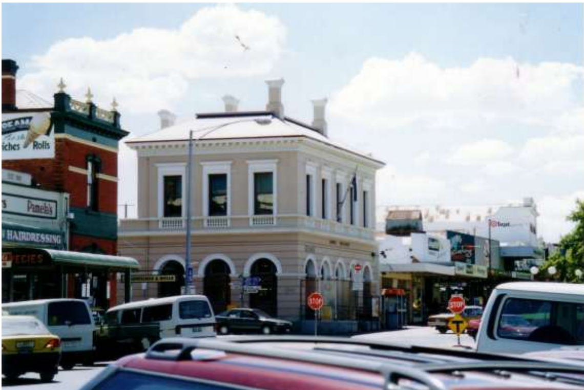
Photo8.0-8: View along Main Street showing introduced shopfronts and parapets, and the early gabled roof forms and monitor roofs (clad in galvanised corrugated iron) behind. The Post Office is visible in the centre. (Source: 'Northern Grampians Shire Heritage Study, Stage 2', 2004)
