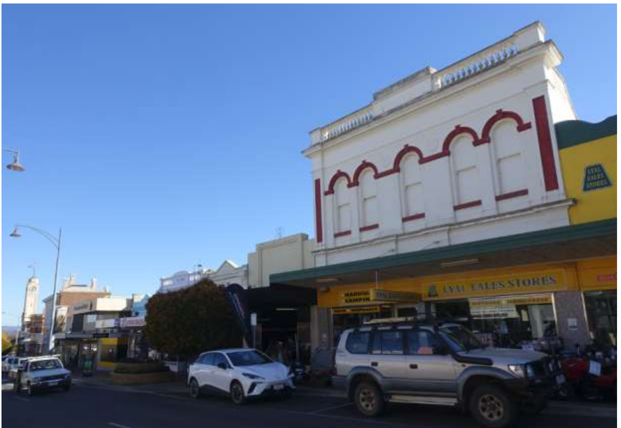
8.18: North side of Main Street, west end, comprising 87-115 Main Street. (Source: Landmark Heritage PL, 2024)
