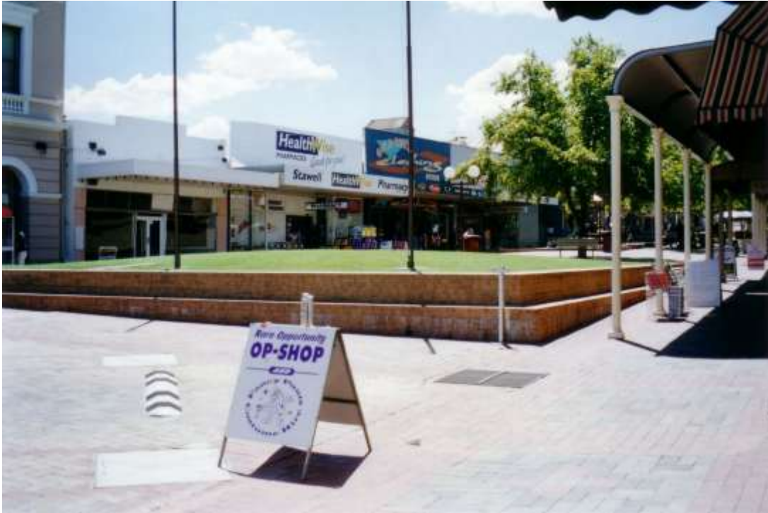
Photo 8.05: Main Street showing new and substantially altered buildings with new shopfronts and over-sizedly proportioned parapets and projecting cantilevering canopies. Note the early roof monitors and gabled roof forms behind some of the introduced parapets. The pedestrian mall has since been removed. (Source: 'Northern Grampians Shire Heritage Study, Stage 2', 2004)
