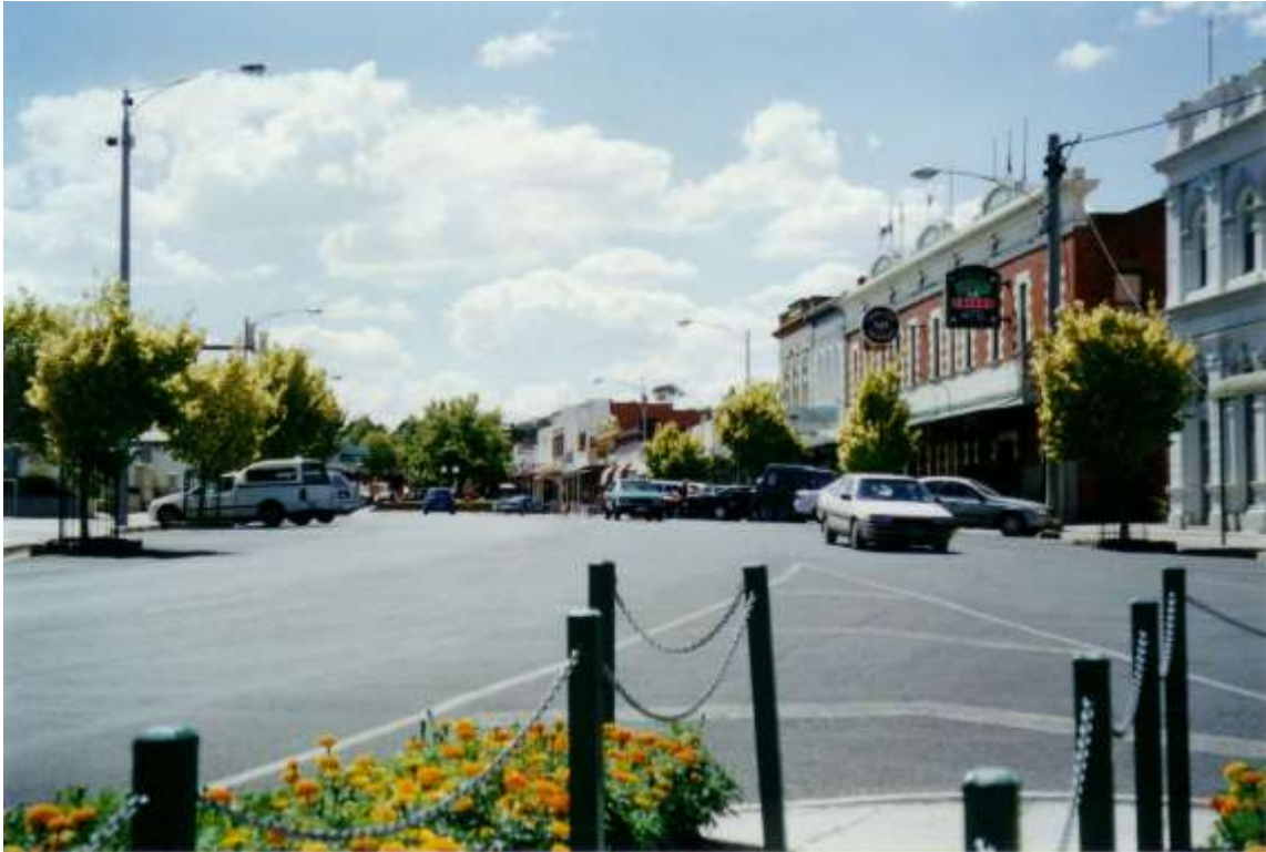
Photo 8.01: Lower Main Street from the War Memorial gardens showing 19 th century Victorian styled two-storeyed commercial buildings. (Source: 'Northern Grampians Shire Heritage Study, Stage 2', 2004)
