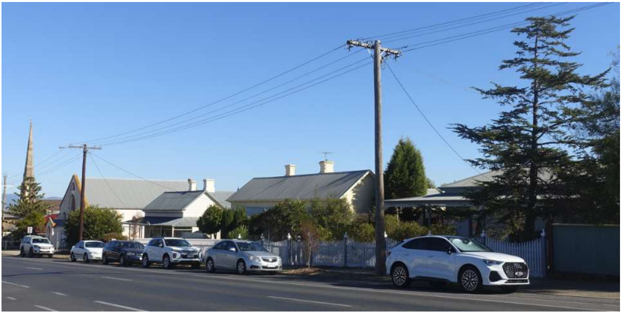
8.26: Victorian houses at 27-31 Scallan Street, looking west. (Source: Landmark Heritage PL, 2024)
