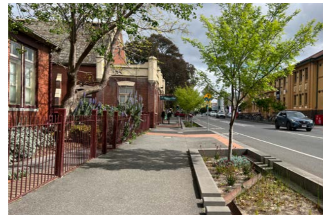
Image 53 Streetscape improvements incorporating WSUD rain gardens on Dawson Street Brunswick
