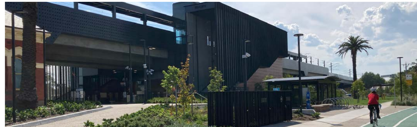
Image 56 Moreland Station has a high visibility from the side streets surrounding, which highlights the presence of the station precinct
