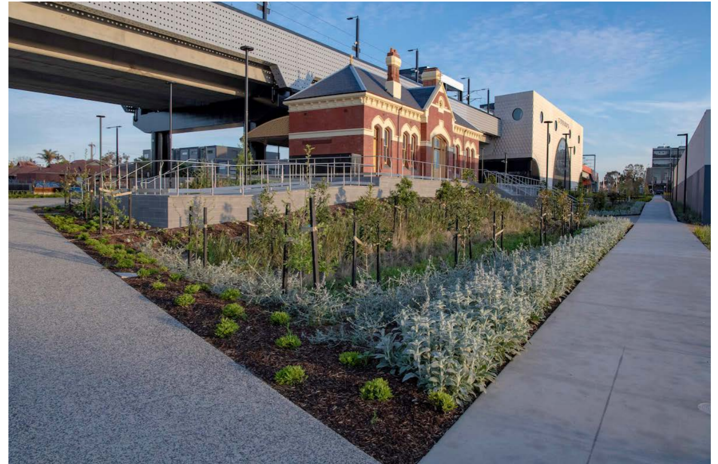
Image 52 Swale with diverse planting mix that is appropriate to the local climate at Coburg Station
