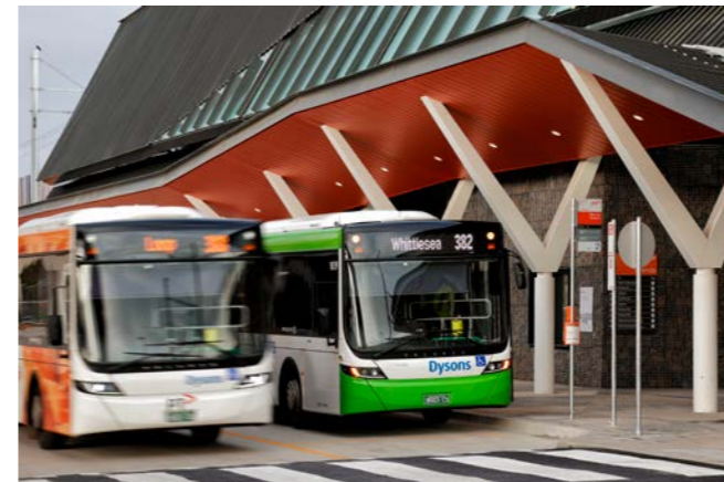
Image 45 Integrated bus stop within Mernda Station precinct
