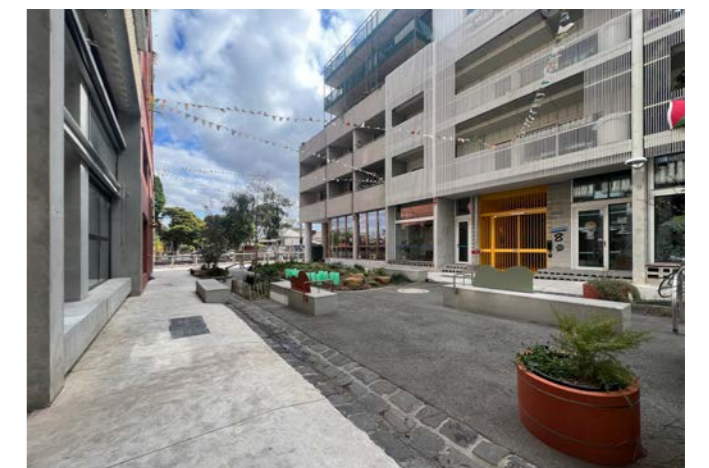
Image 33 Shared path and rail corridor at the end of Duckett Street surrounded by high-density residential and mix uses developments.
