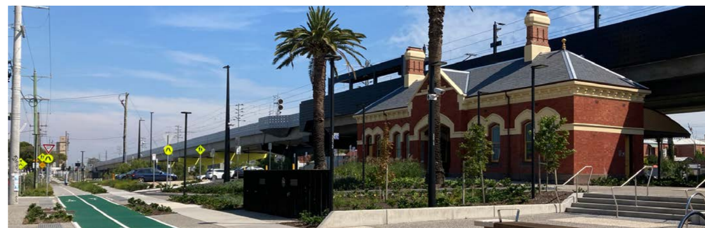
Image 35 Moreland Station building re-purposed and integrated into the corridor to maintain and celebrate the historical character of the site
