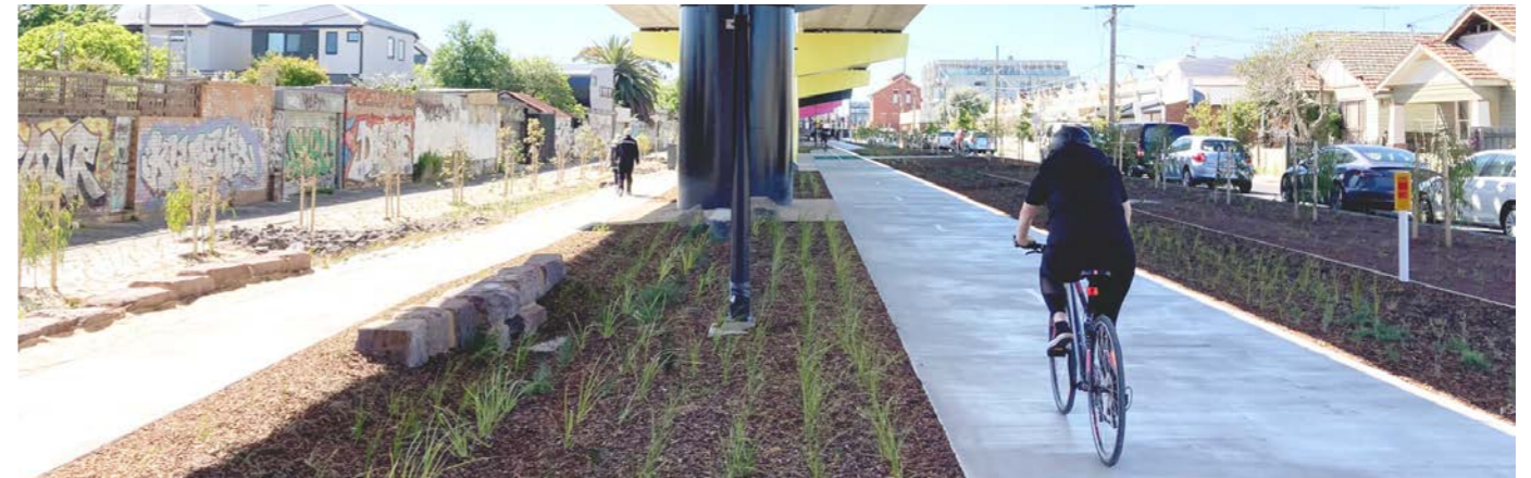
Image 44 Bell to Moreland separated cyclist and pedestrian path
