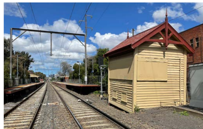
Image 8 Victoria Street signal box at Brunswick Station
