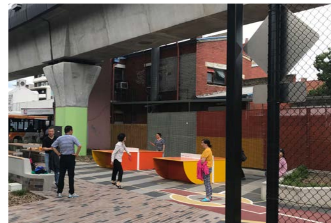
Image 41 The design of the open space adjacent to Carnegie Station responds to the current needs of the community and future urban growth
