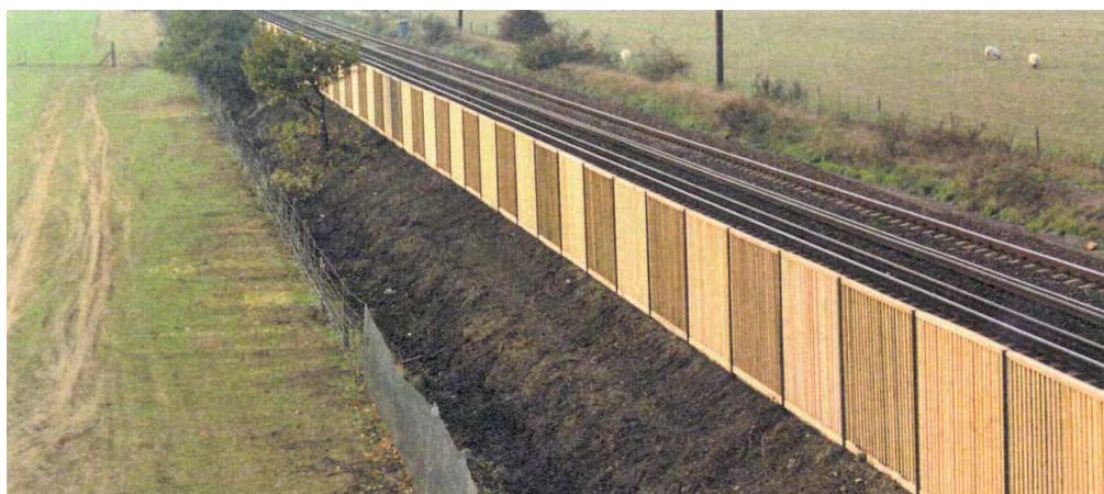
Figure 1: Typical timber wayside noise barriers adjacent to railway.
