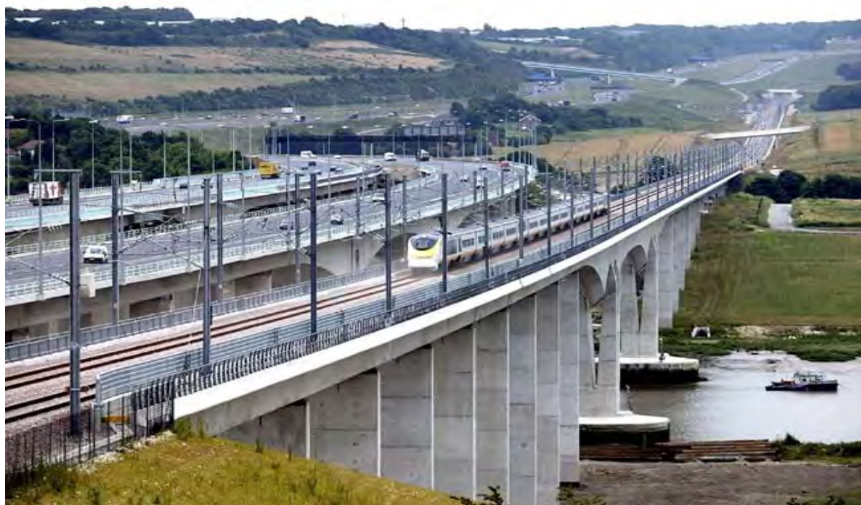
Figure 2 Low-level trackside noise barriers on Medway Viaduct, UK.
