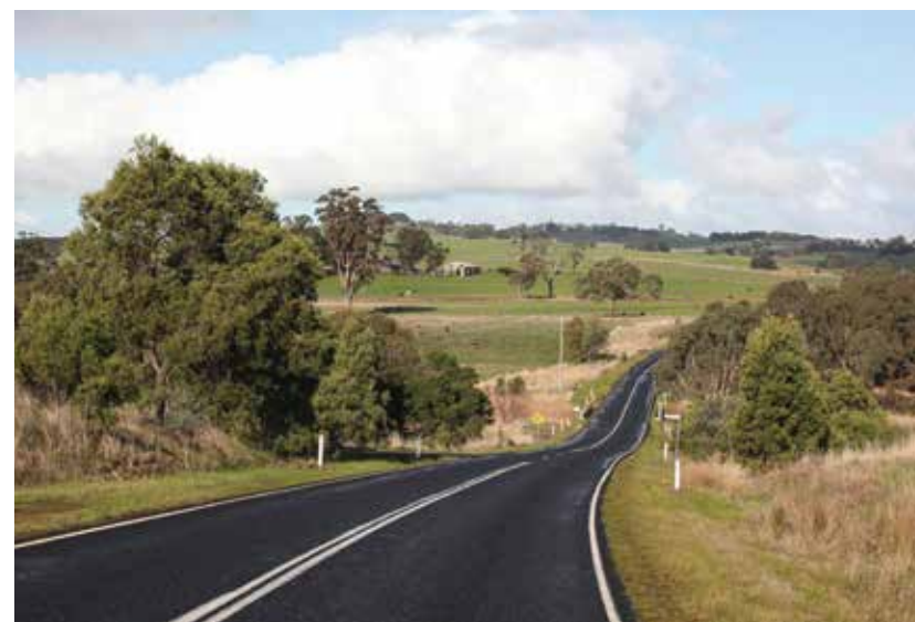
Rural road near Sandford, Glenelg Shire
