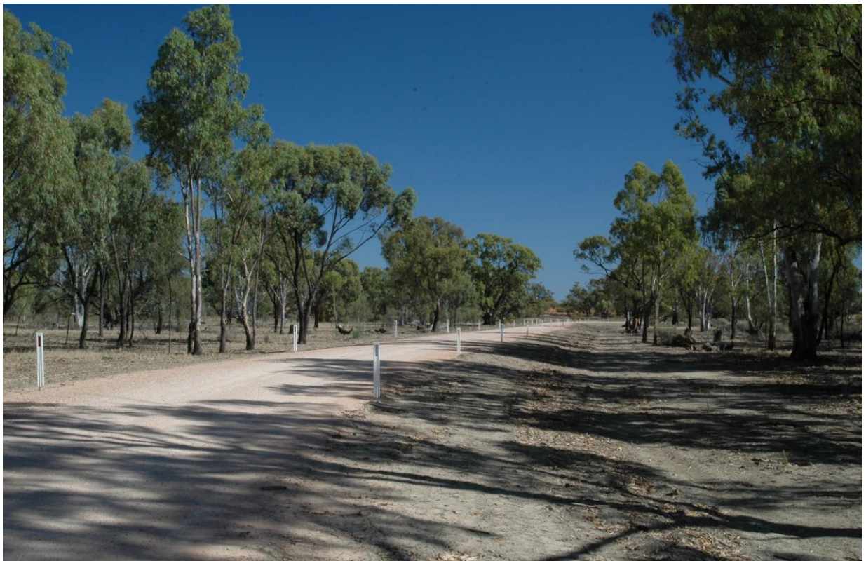
Figure 5 – A containment bank constructed under The Living Murray at the Hattah Lakes, similar to those proposed for Vinifera
