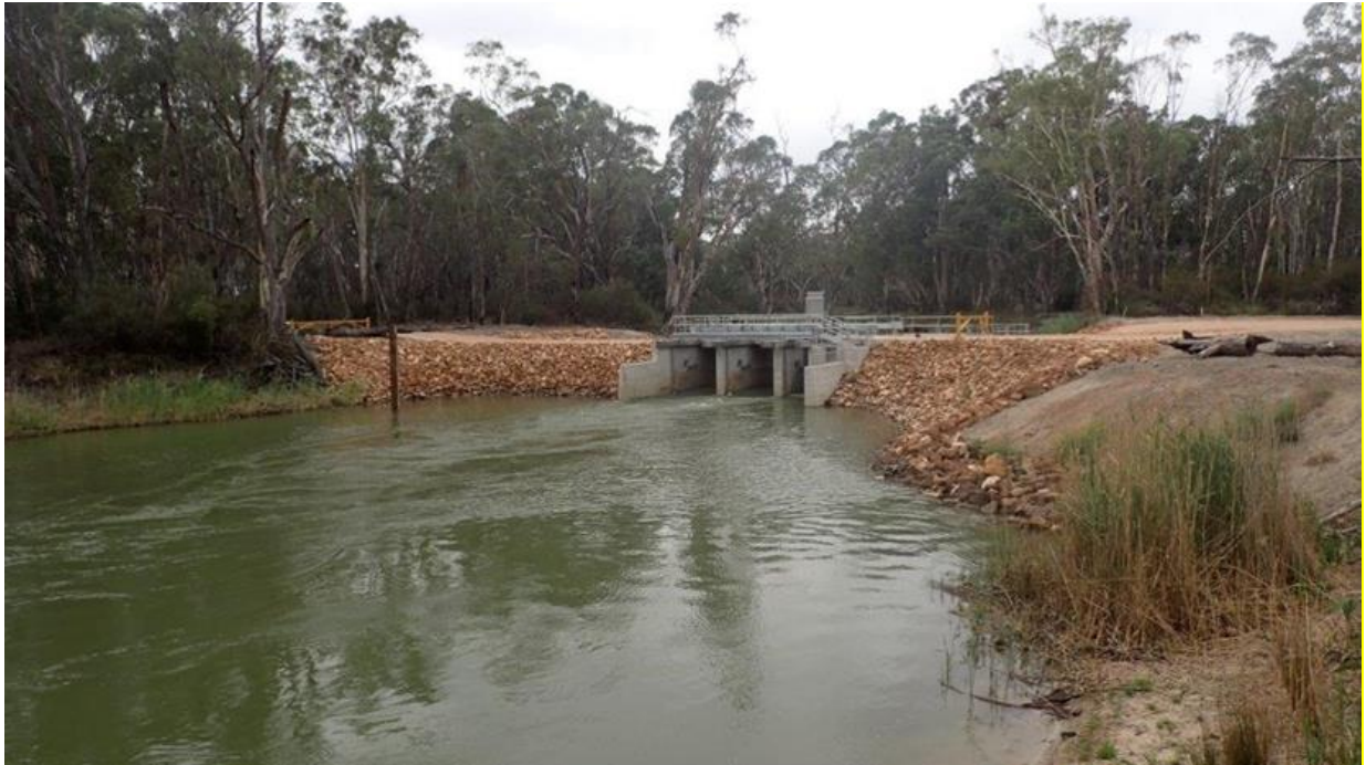
Figure 4 – A regulating structure at Mullaroo inlet (Lindsay Island), similar to the proposed regulator V2 and V1
