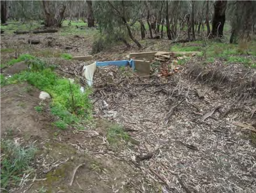
Figure 8 Nyah channel weir
