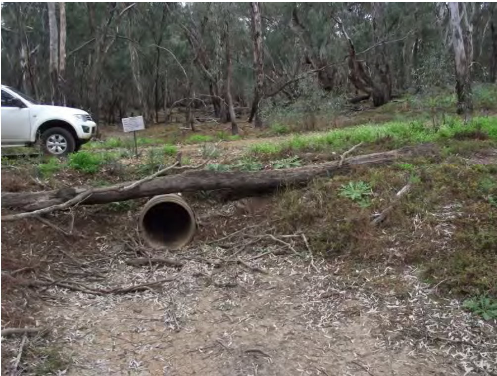
Figure 9 Culvert at Downstream End of Parnee Malloo Channel
