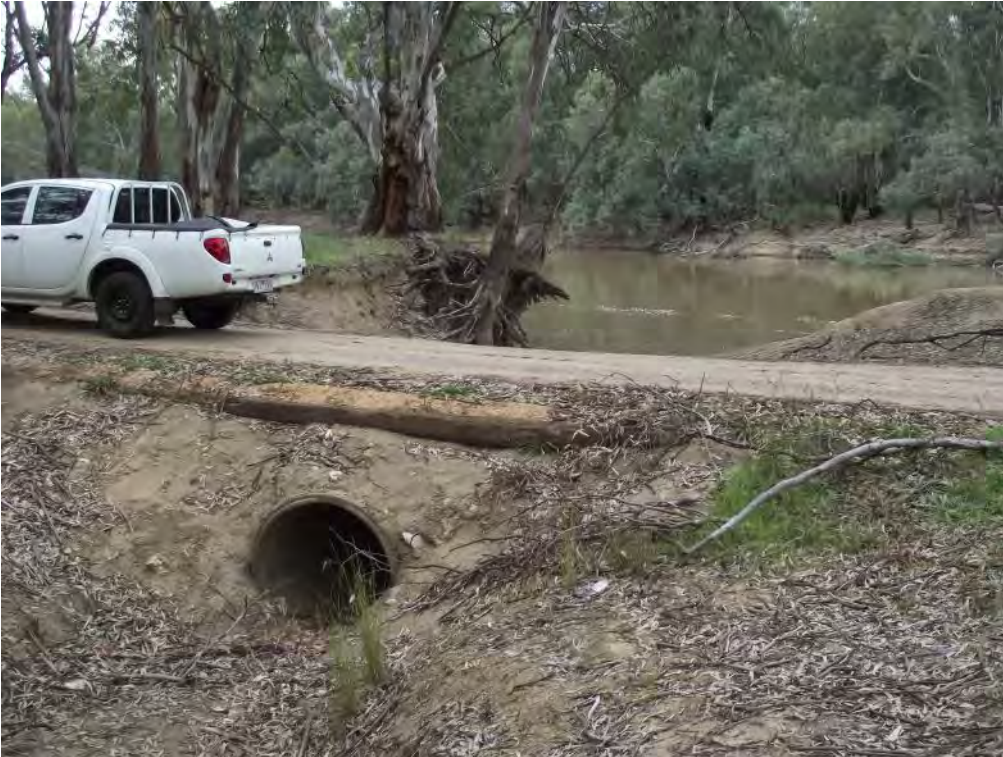
Figure 7 Culvert at upstream entrance to Nyah Channel
