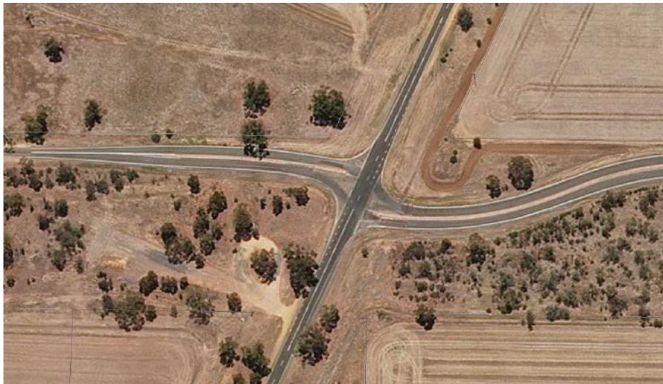
Figure 1 – Key Intersection 1 – Henty Highway and Minyip-Dimboola Road
