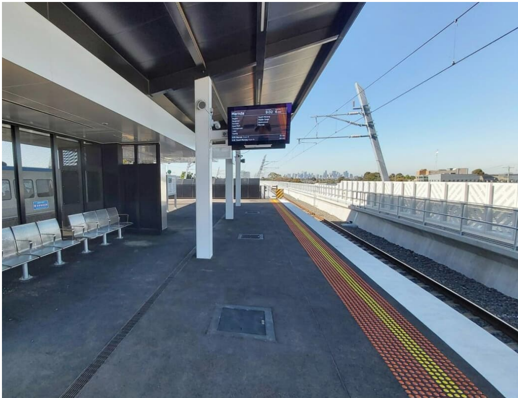
Figure 11 Preston Station privacy screening with normal height rail bridge screening in the distance
