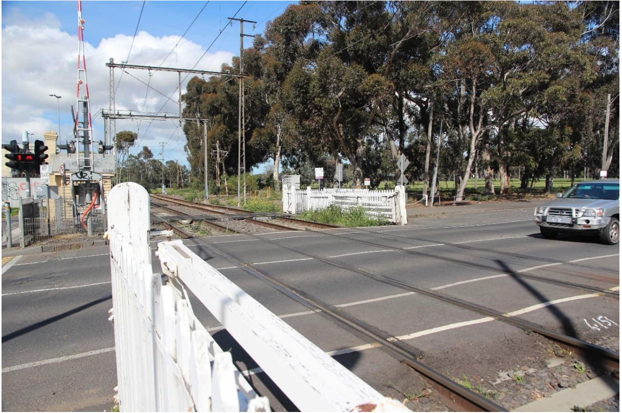
Figure 6 Park Street Level Crossing with Royal Park to the south and heritage listed elements in background (signals pole and signals hut)
