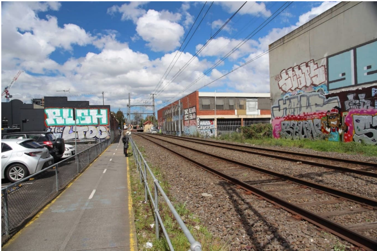
Figure 7 Upfield Rail Corridor – north of Victoria Street, looking back to Brunswick Station. Upfield Shared path with light industrial sites to the east and west of the corridor
