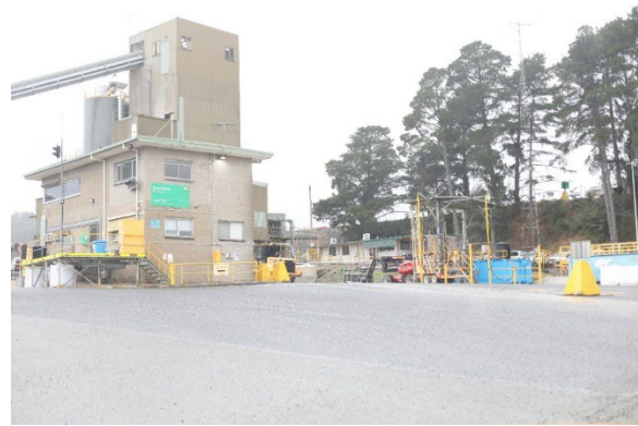
Image 4: Processing Area 2 – Concrete
