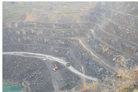
Image 6: Existing Haul Road into the Pit
