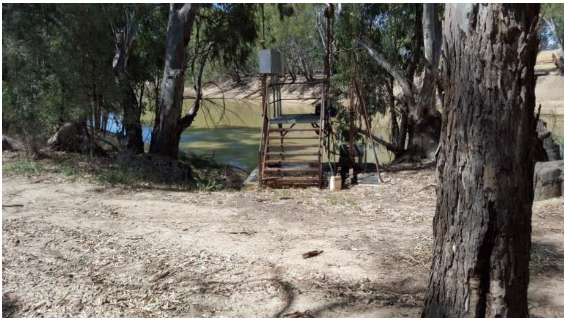
Figure 15: Existing private pump station adjacent to proposed temporary pump hardstand and Spillway 4
