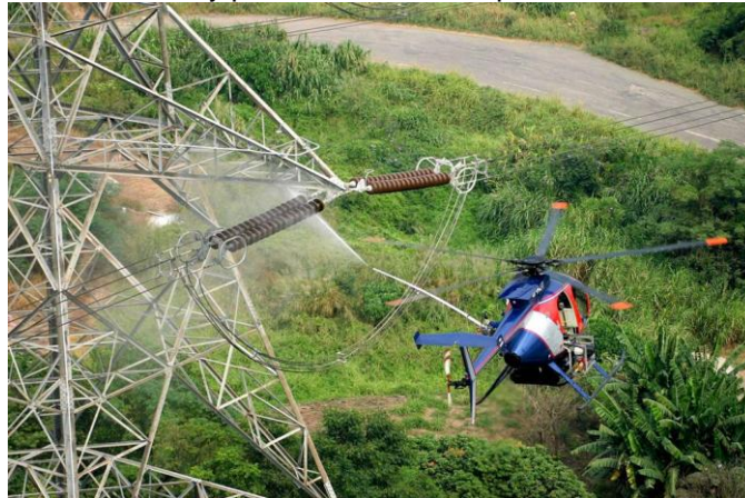
Washing insulators using a MD 500 helicopter.
