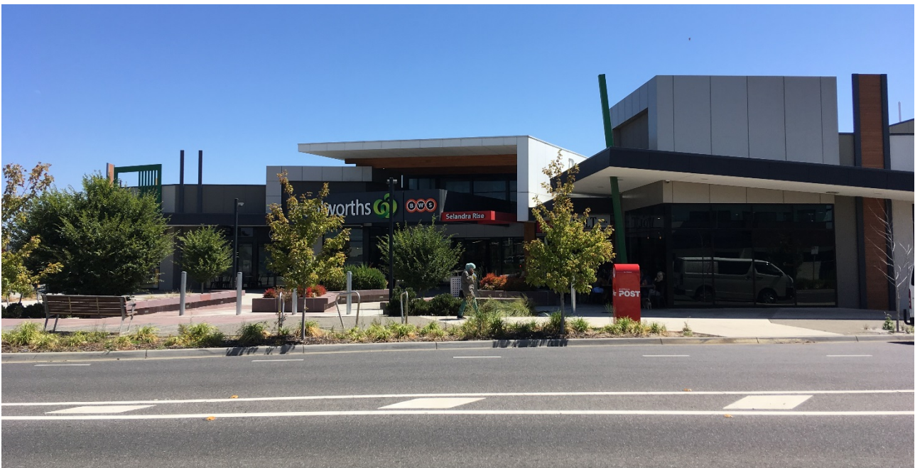
Figure 17: Shopping Centre in Selandra Rise
