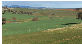
The same pipeline easement, after reinstatement.
