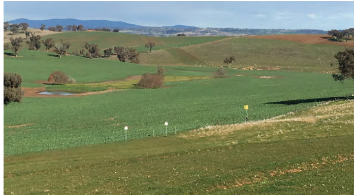
The same pipeline easement, after reinstatement.
