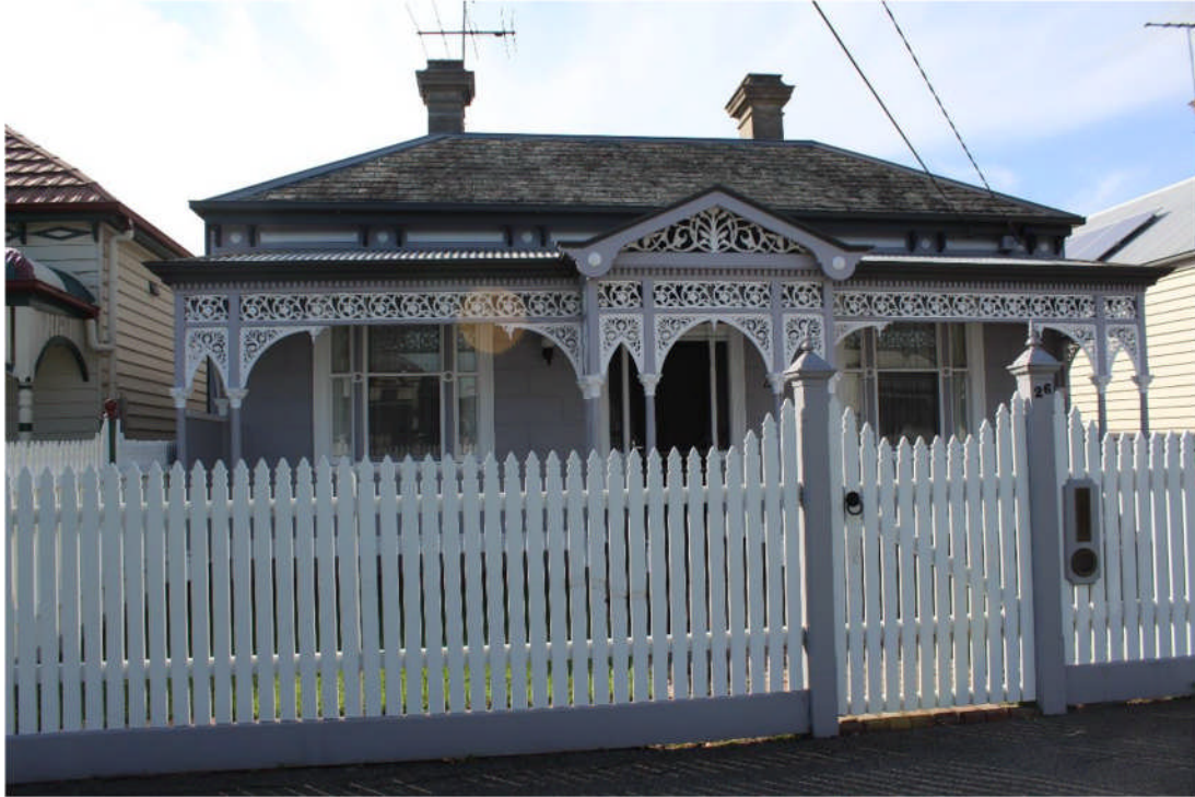
26 Roseberry Street, Ascot Vale, principal elevation (April 2018) (source: Context, 2018)
