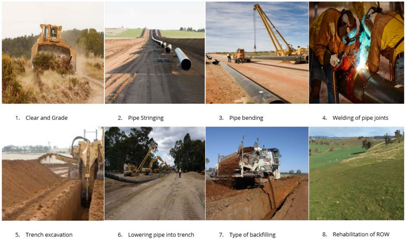
Figure 1 Pipeline construction phase
