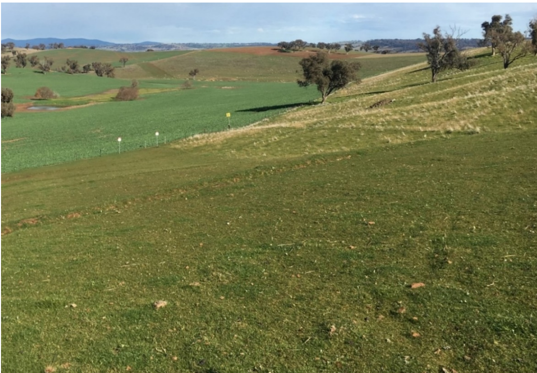
Figure 4: ROW approximately 7 months after construction (July 2017)
