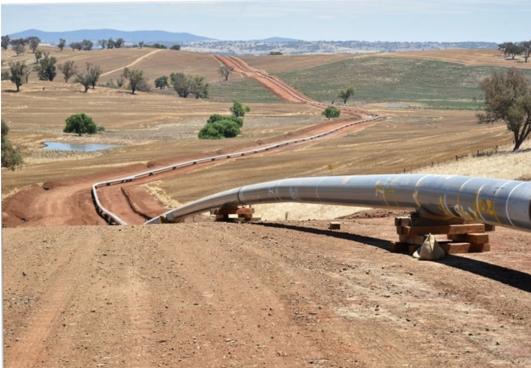
Figure 3: ROW during construction (Jan 2017)
