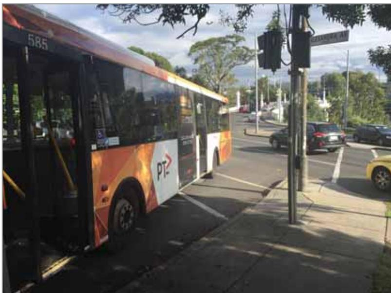
76. The example above should not be occurring and can be easily fixed (particularly given there are only peak period clearways in this segment of Punt Road). It only occurs due to carriageway geometry that seems to make provision for a triangular vehicle to pull into the kerb south of Alexandra Avenue as shown in Figure 5 below. If a full size bus comes any further forward than that shown in Figure 4 then the front of the bus will stick out into the left hand traffic lane.
