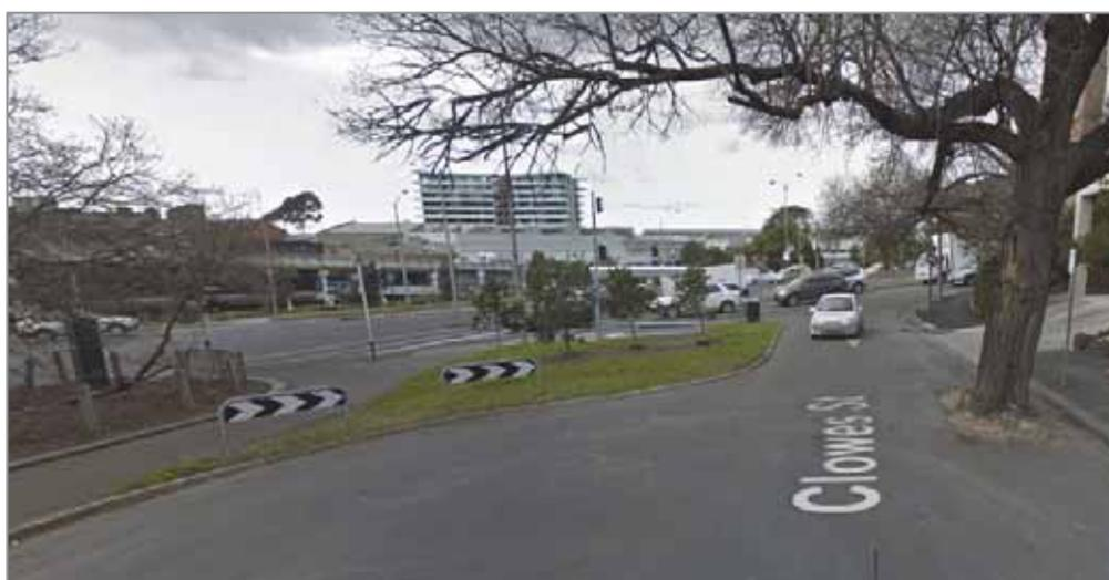
182. As an example of how minor changes can help to avoid Braess Paradox occurring, Clowes Street could be fully closed at Punt Road. This would result in slightly less traffic queuing in the northbound lanes at the Alexandra Avenue intersection and require drivers to find an alternative path into Clowes Street (from Anderson Street). The reduction in vehicles on Punt Road would be equal to (or slightly more than) the number of drivers inconvenienced by the change.
