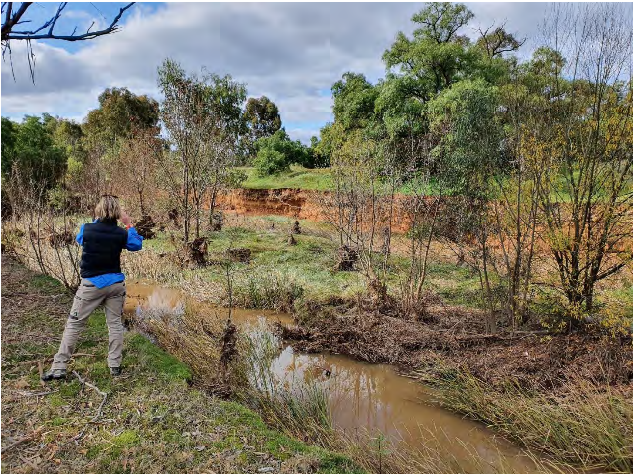
FIGURE 3-7 DOWNSTREAM VIEW OF BENDIGO CREEK WHERE CHANNEL WIDENING HAS OCCURRED.
