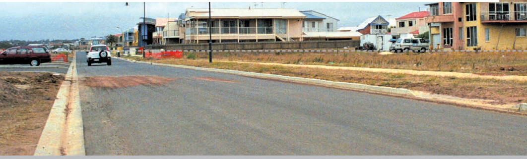
ABOVE | The sprawling eastern edge of Torquay
