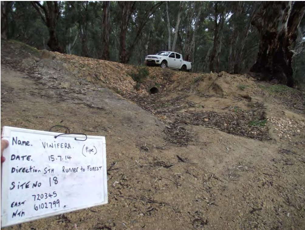
Figure 8 Existing Culvert at 720345 E 6102799 N
