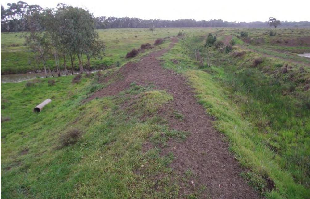
Figure 9 Levee and Irrigation Channel at 721610 E 6102848 N
