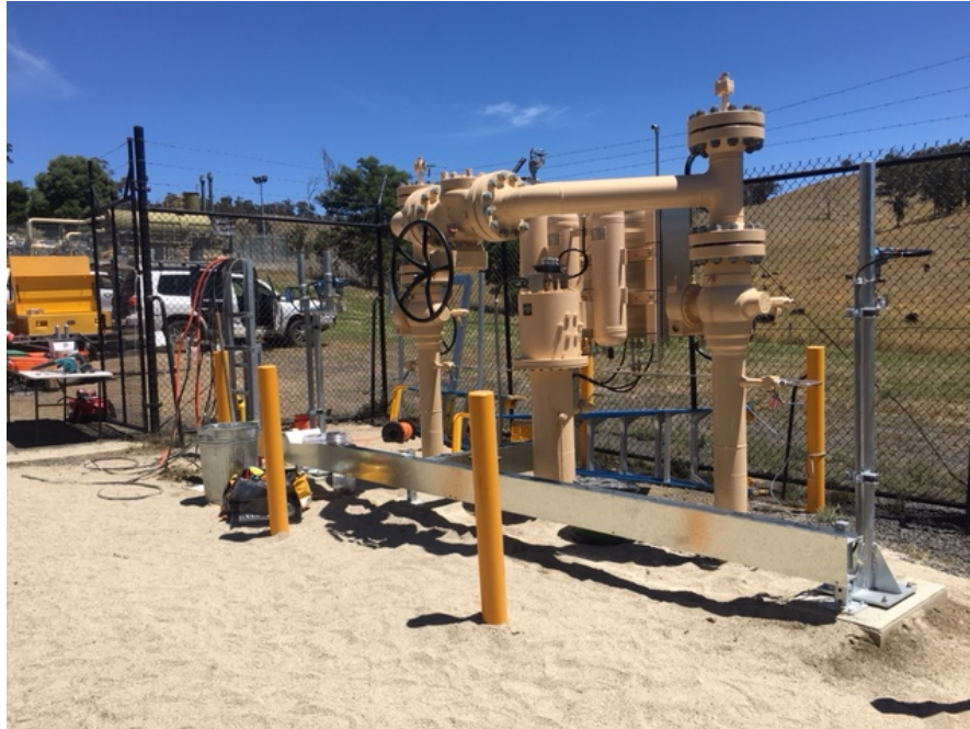
Figure 6 Typical layout of a mainline valve
