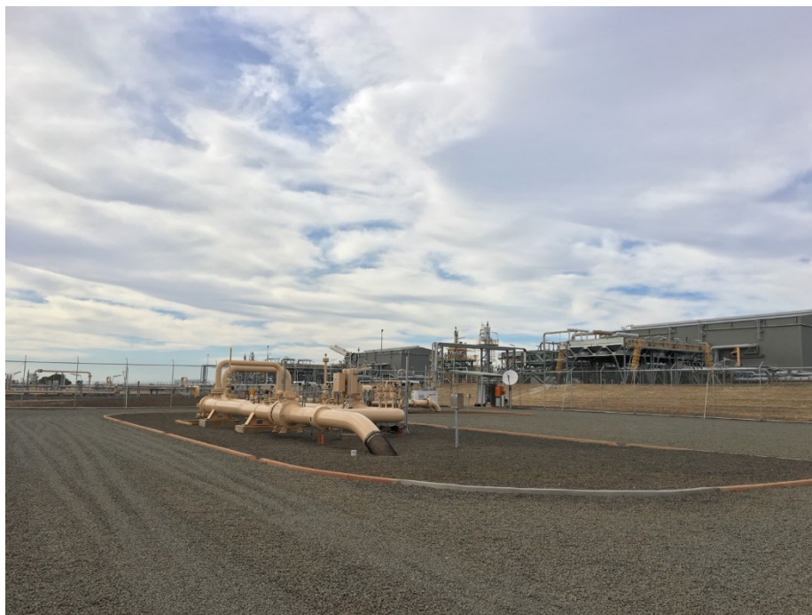
Figure 5 Typical layout of a scraper station
