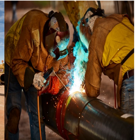
4. Welding of pipe joints
