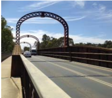
Photo 2: The existing bridge
