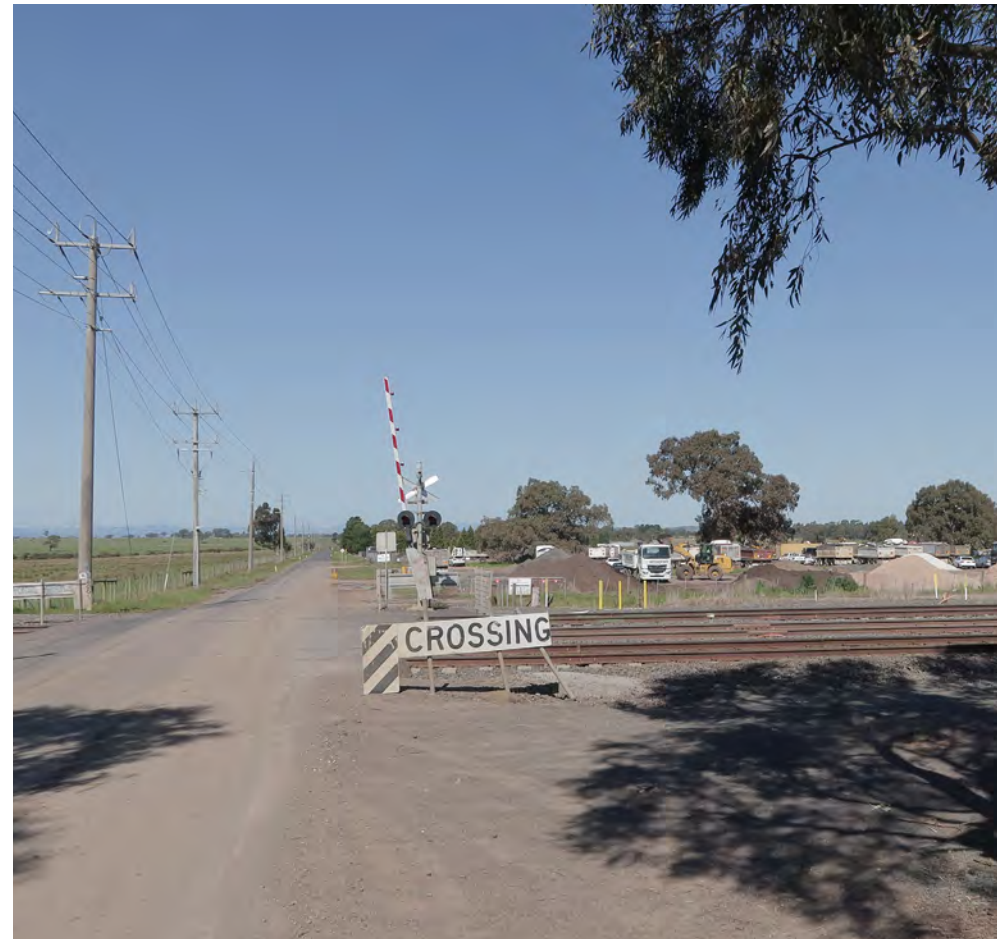
FIGURE 11 RAILWAY CROSSING AT SUMMERHILL ROAD
