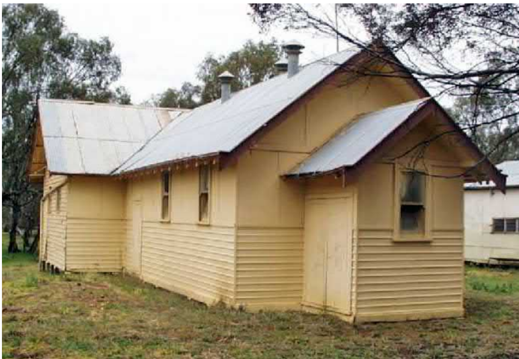
Figure 2.7: Former Church (HO201), located within the Kulki Kulki Scout Camp (Allom Lovell and Associates 2001c, p. 551)
