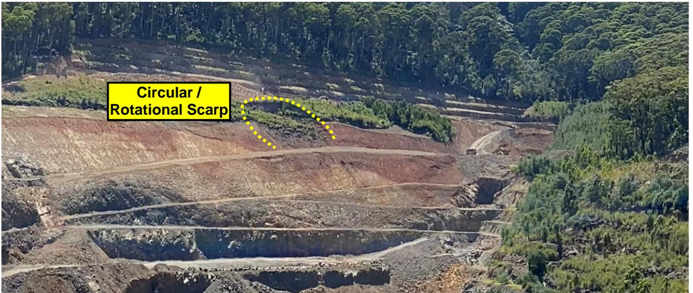
**Figure 27** *Photograph Depicting Circular/Rotational Type Instability – Northern Wall*
