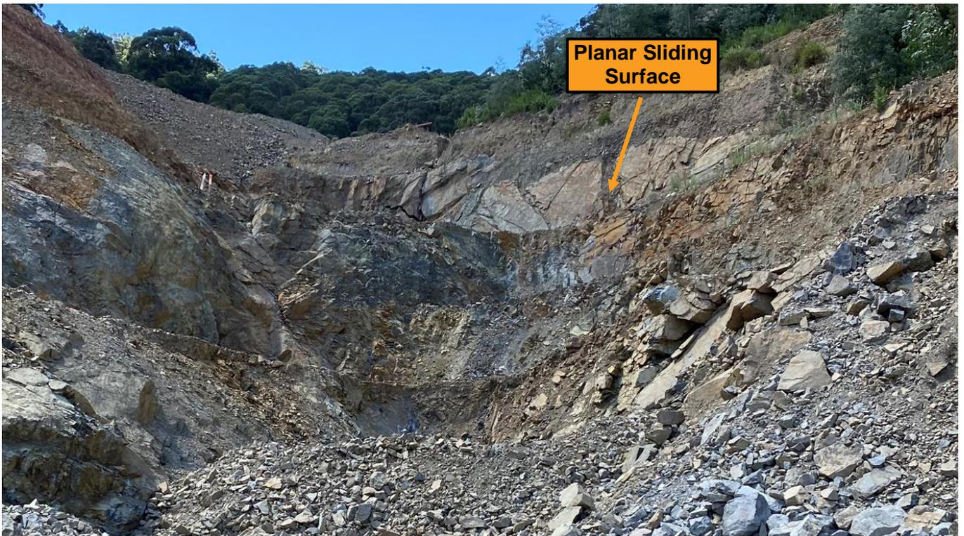
Figure 22 Photograph Depicting Planar Sliding Surface – North East Corner
