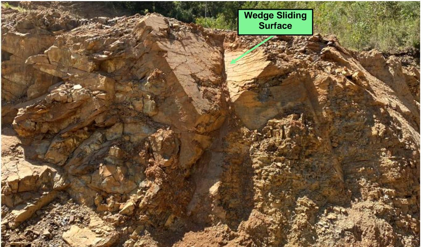
Figure 23 Photograph of Minor Wedge Formation – Northern Corner
