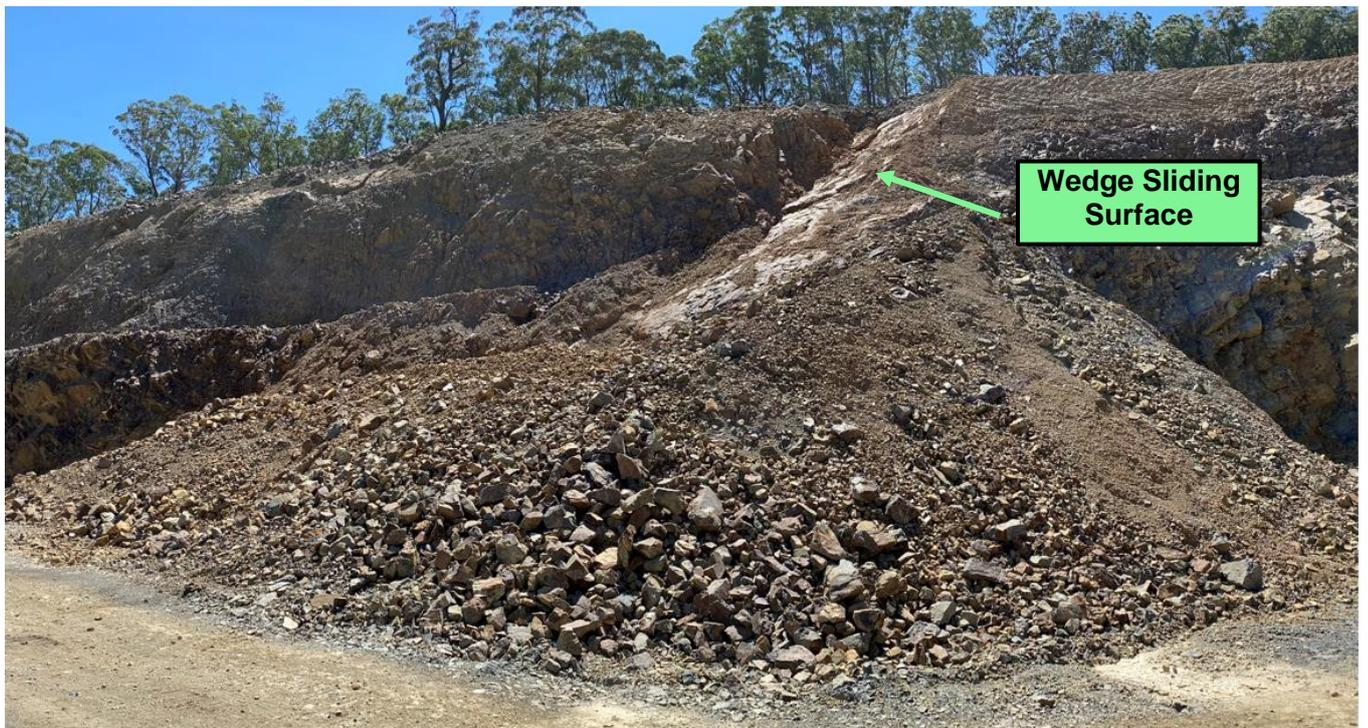
Figure 24 Photograph of Minor to Moderate Wedge Formation – Northern Corner
