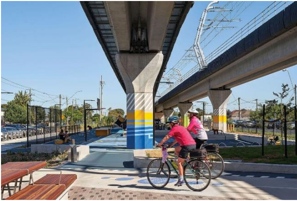
Figure 9.5 Single piers with a slender super-T girder and coloured base (image: Caulfield to Dandenong).
