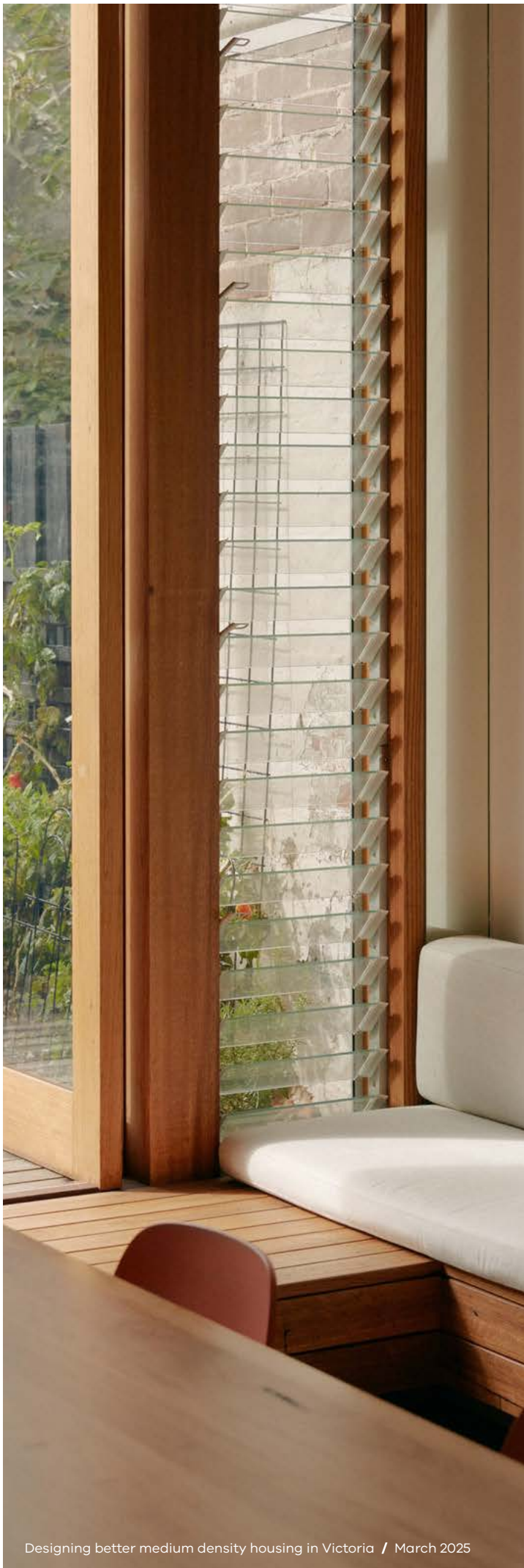
◀ Figure 69. Internal louvres can allow occupants to effectively manage natural ventilation.
