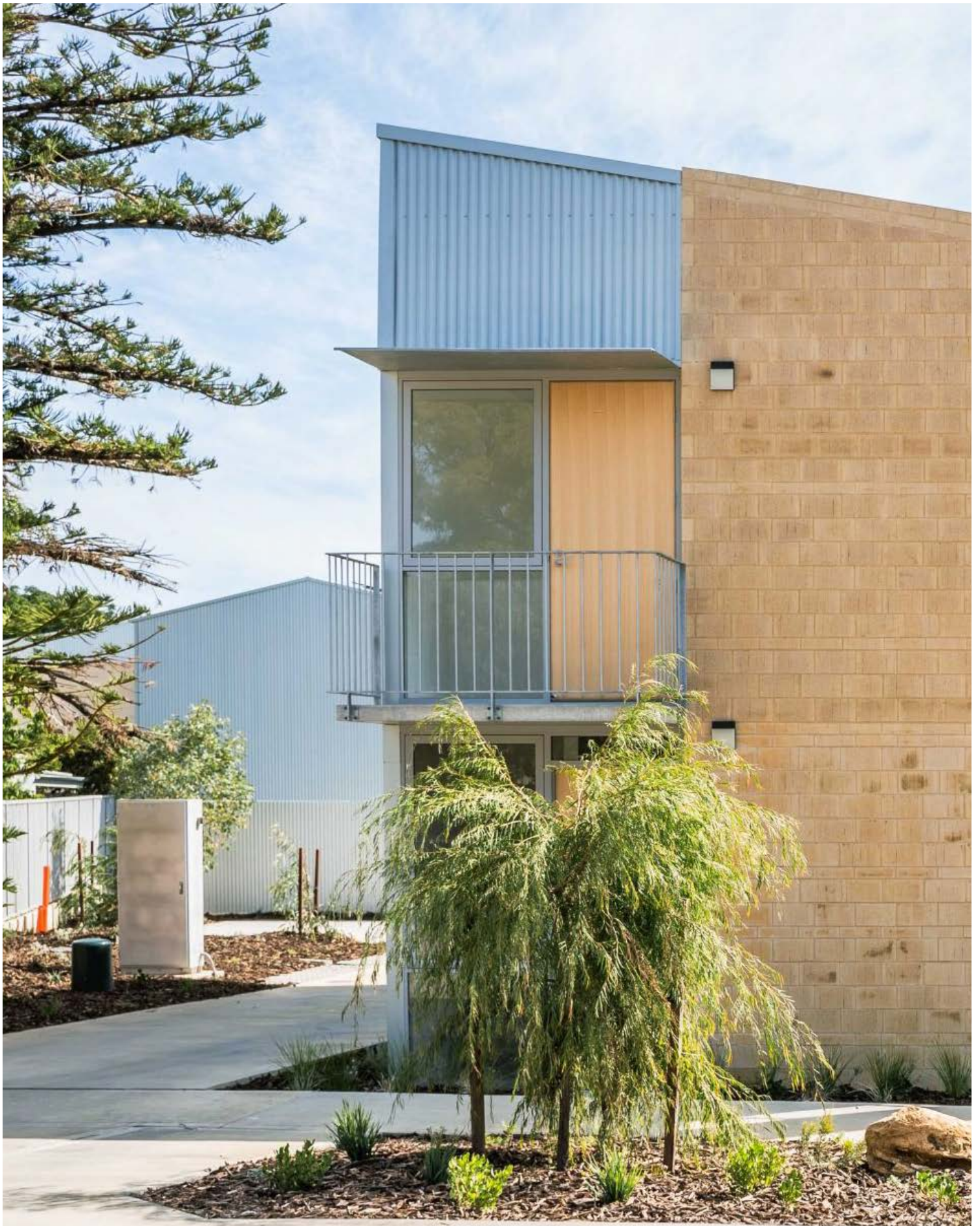
▲ Figure 79. Considered use of durable and robust materials with quality detailing. The material choice suits the local area and climate conditions, and the facade has been designed for low maintenance.
