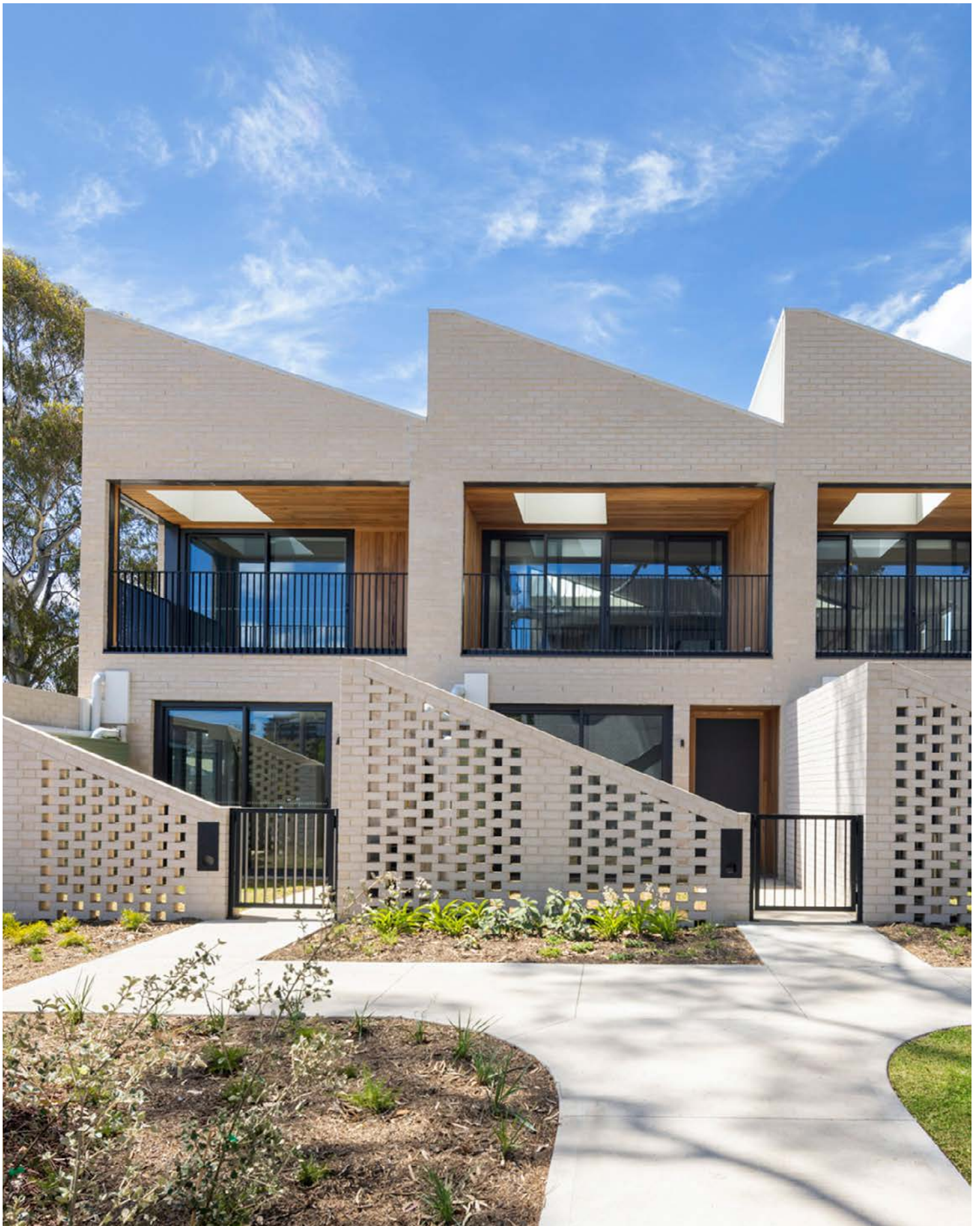
▲ Figure 37. Compact water tanks used for rainwater harvesting are tucked behind brick screens to minimise their visual impact across the facade.
