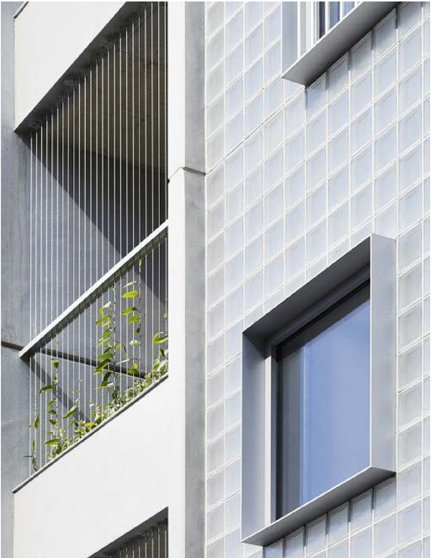
▲ Figure 76. Balustrades with built in planter boxes and cables. Light Box, Collingwood, VIC / Clare Cousins / Photographer: Tess Kelly
