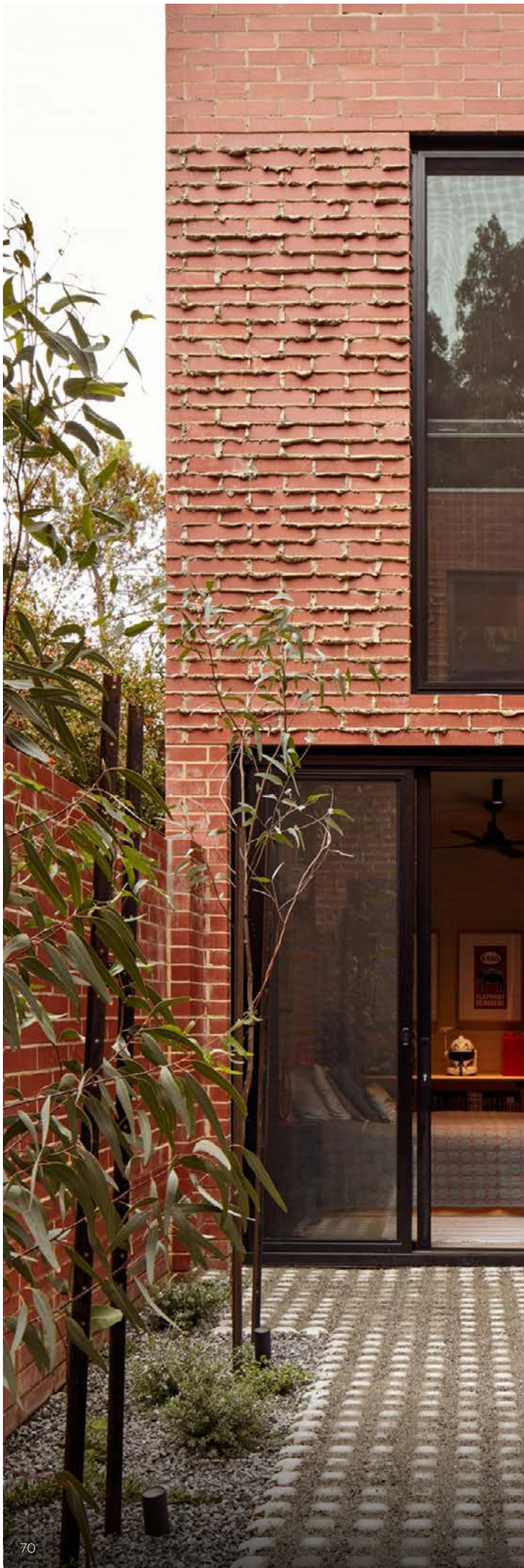
◀ Figure 46. Permeable ground surface covers include lawn, mulch and garden. Use ground cover planting where possible.
