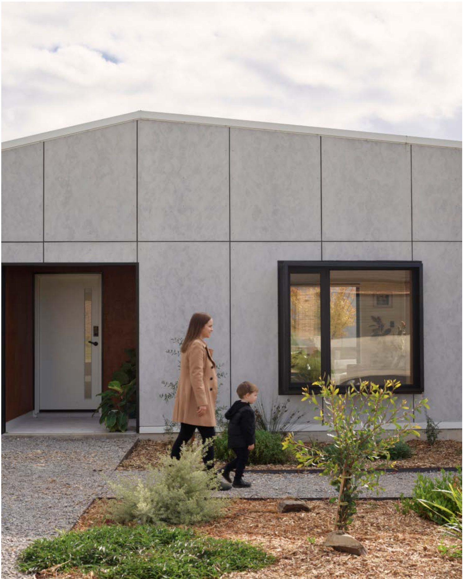
▲ Figure 92. Fibre cement (FC) sheet cladding is highly energy efficient, sturdy and contains fire-resistance properties. Avoid using FC sheet with an applied paint finish where possible, as this will increase the need for ongoing and regular maintenance.
