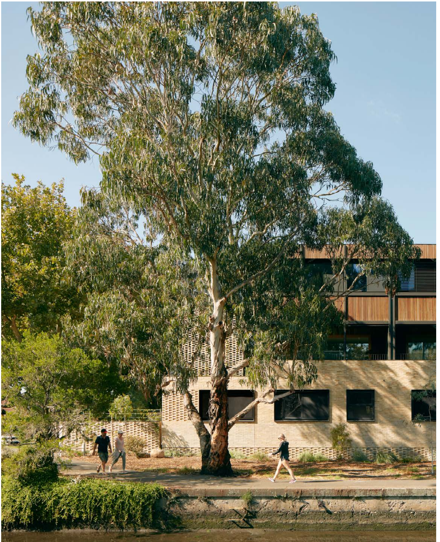
▲ Figure 1. The design of this townhouse development addresses the site's boundary conditions between a residential area and a canal. The scale, setback and materiality of the residential facing frontage responds to its domestic context, while the northern interface addresses the canal-edge. A landscape buffer between the development and shared path provide privacy to dwellings.
