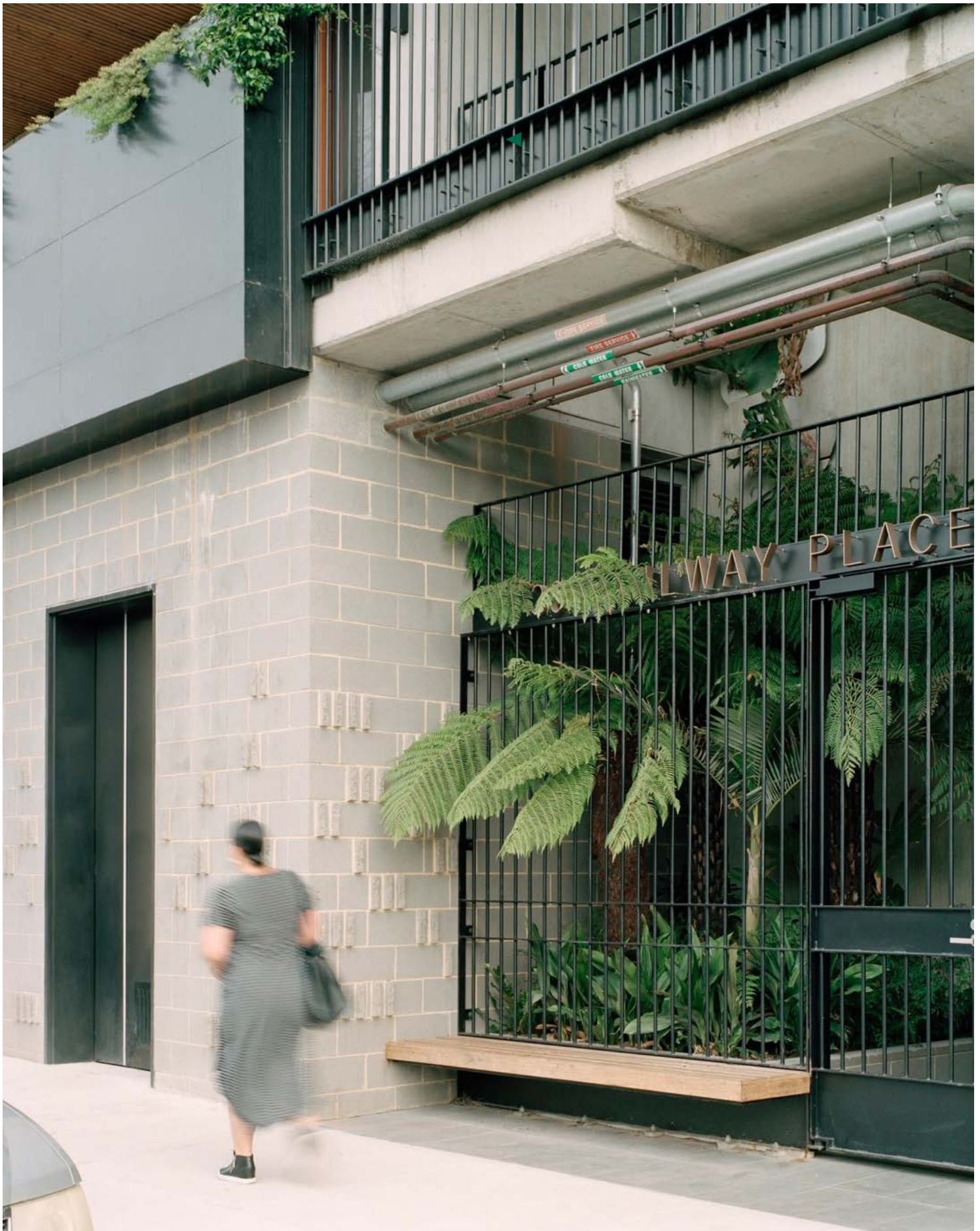
▲ Figure 95. Exposed blockwork with protruding details on the ground floor wall creates visual and tactile interest. The solid concrete block wall is complemented by softer elements like timber seating and lush plants.
