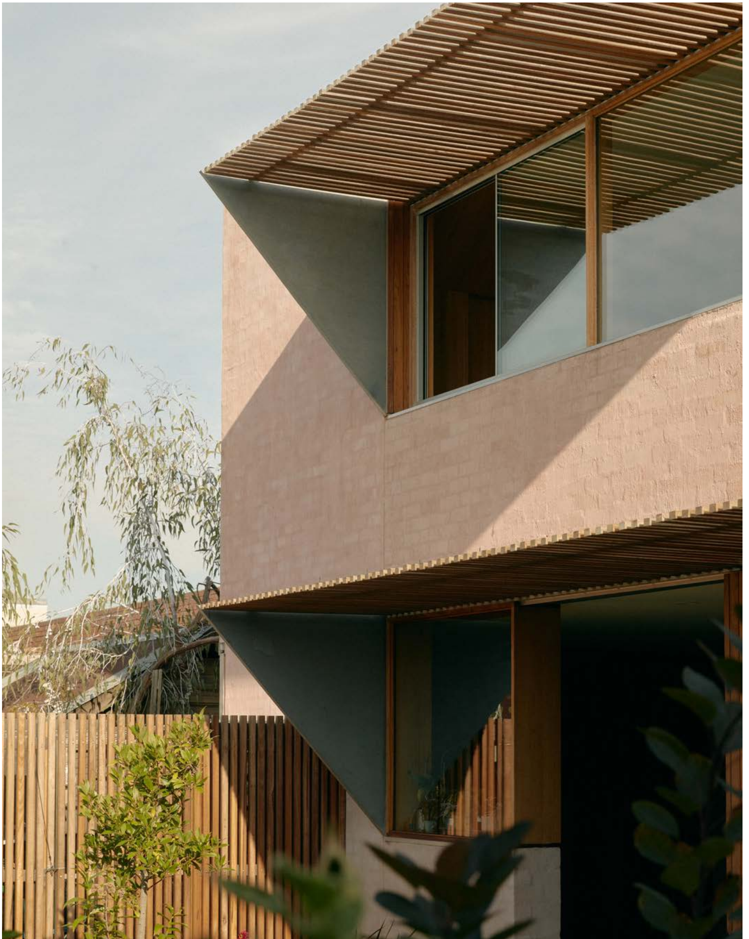
▲ Figure 84. Timber battens can provide shading that does not look overly dominant, while still allowing light to penetrate.
