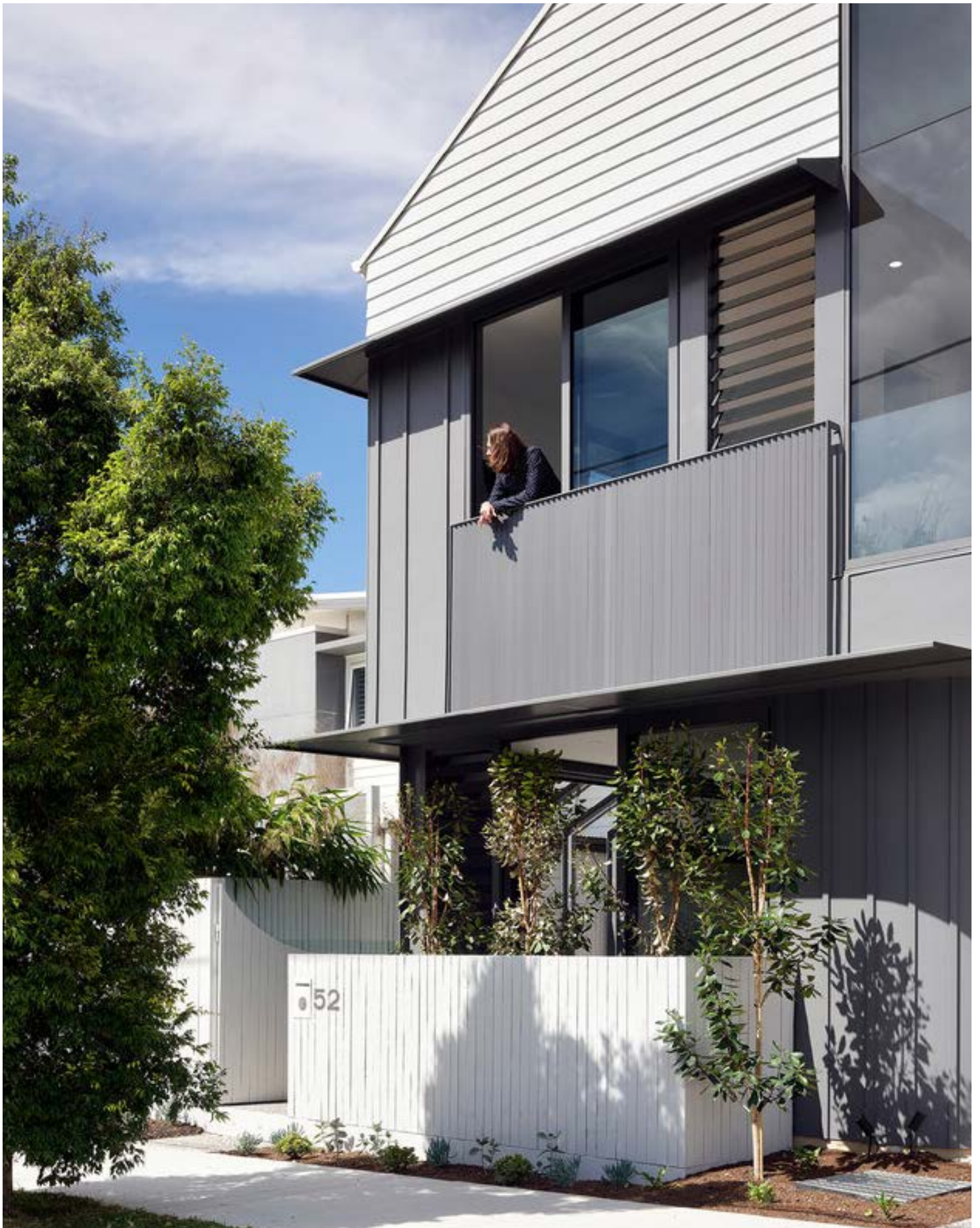
▲ Figure 4. This townhouse development is carefully sited to maximise outlook directly to the street, with a legible building entry, upper level balcony and garden facing the street.
