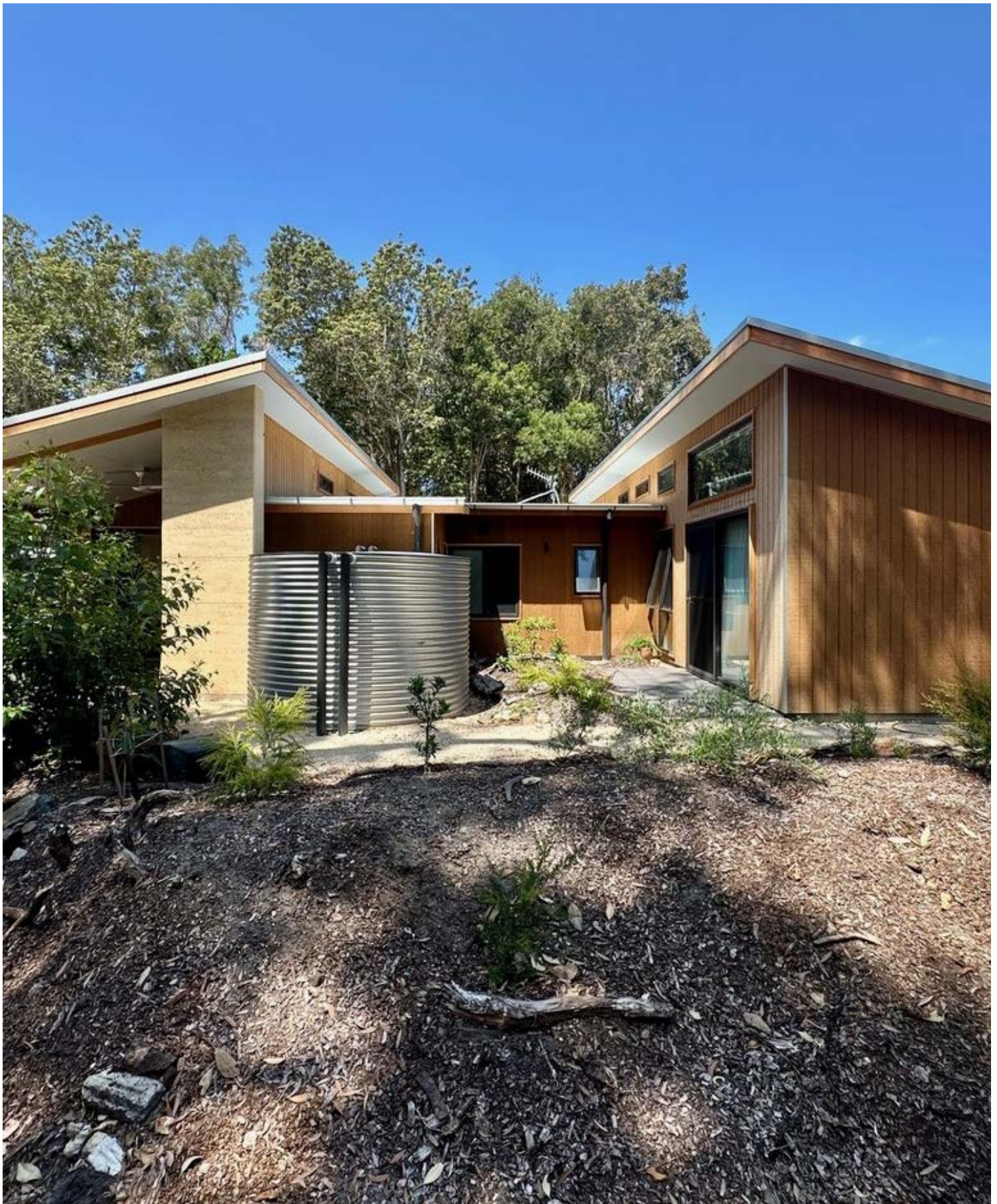
▲ Figure 104. This largely energy-independent building uses light colours and natural materials such as rammed earth for high thermal mass. Windows from west to east allow winter sunlight to warm the southern interior and provide ventilation in the summer. The design optimises passive solar heating, maximises PV power generation and uses battery storage, minimising energy used for heating and cooling. Water conservation is integral to both the building and the garden.
