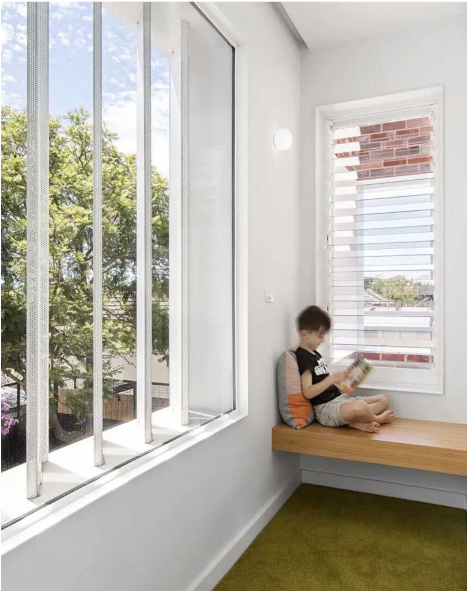
▲ Figure 22. Angled perforated metal fins used to direct views outward. Elsternwick House / Clare Cousins Architects / Photographer: Lisbeth Grosmann
