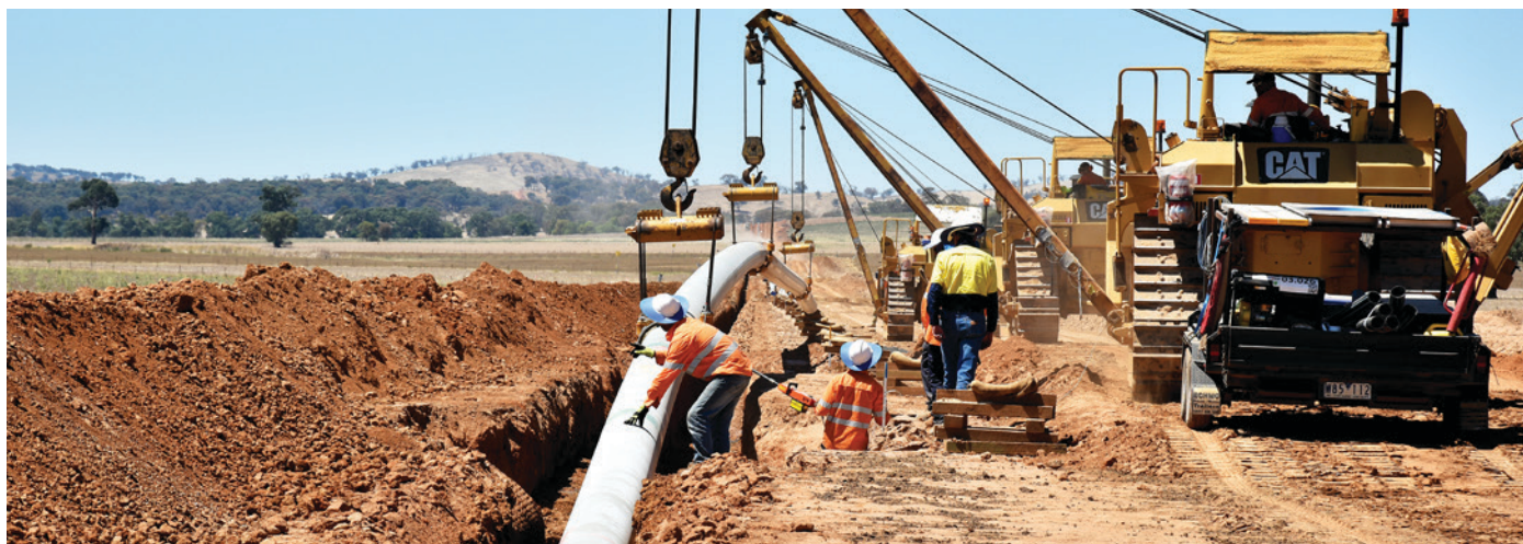
Figure 9: An example of pipeline construction carried out by APA, January 2017.
