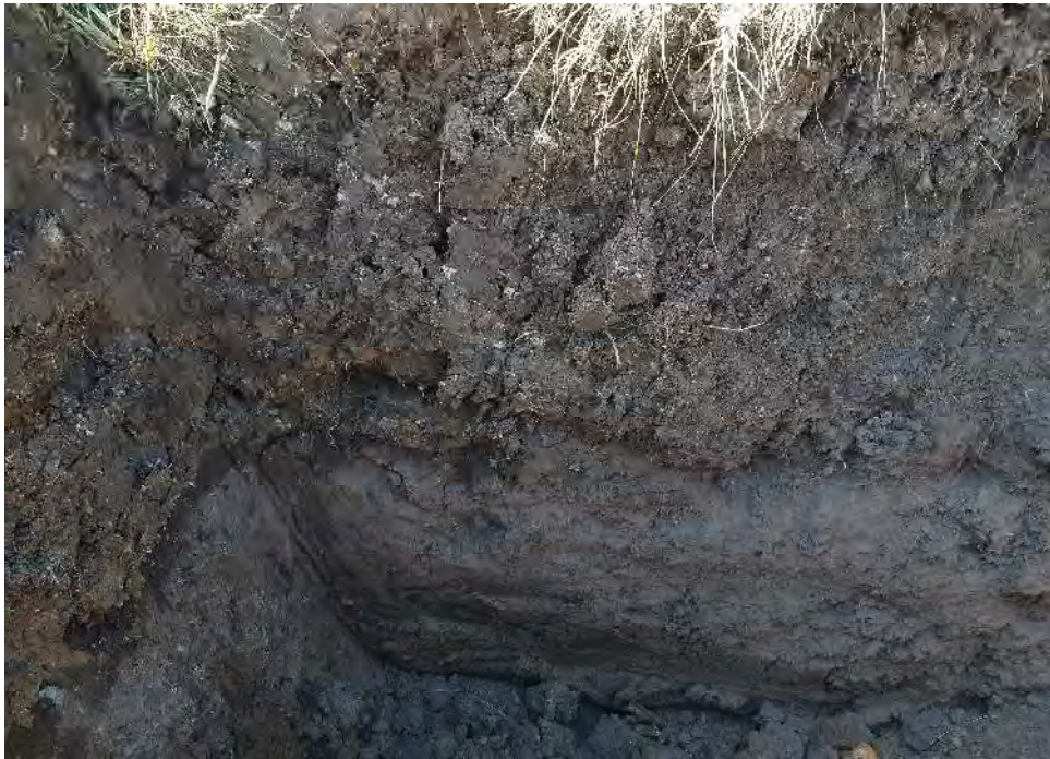
Photo 4 – Fill overlying natural clay (Test Pit TP24)
