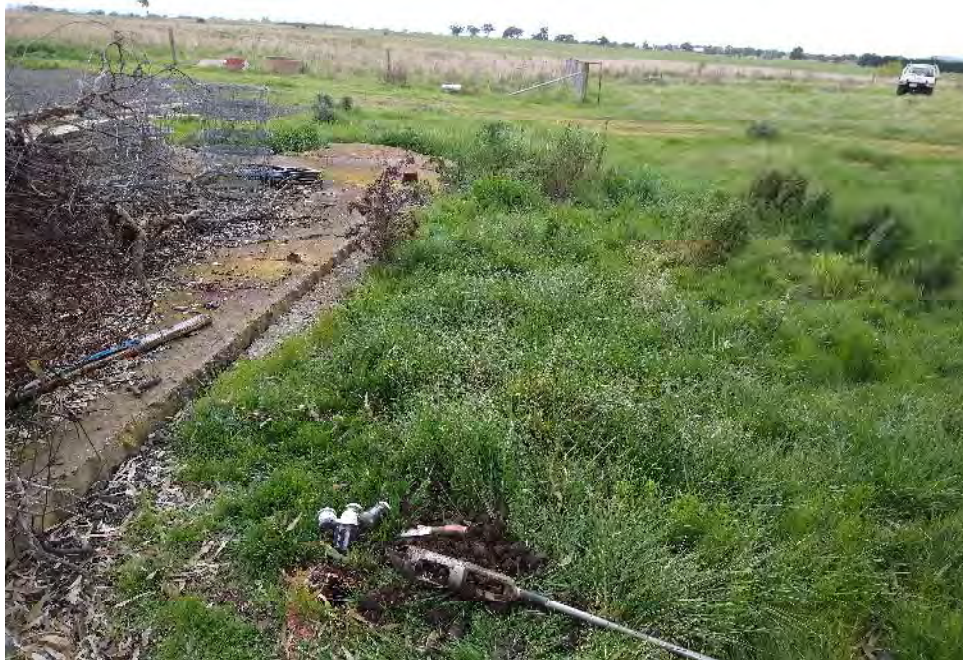
Photo 3 – View edge of former building footing and HA03 (view to the east)
