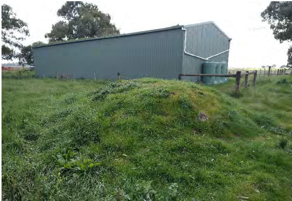
Photo 1 – View of main shed with stockpile in foreground (View to the north-east)
