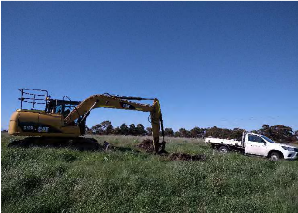
Photo 5 – Typical test pit operation
