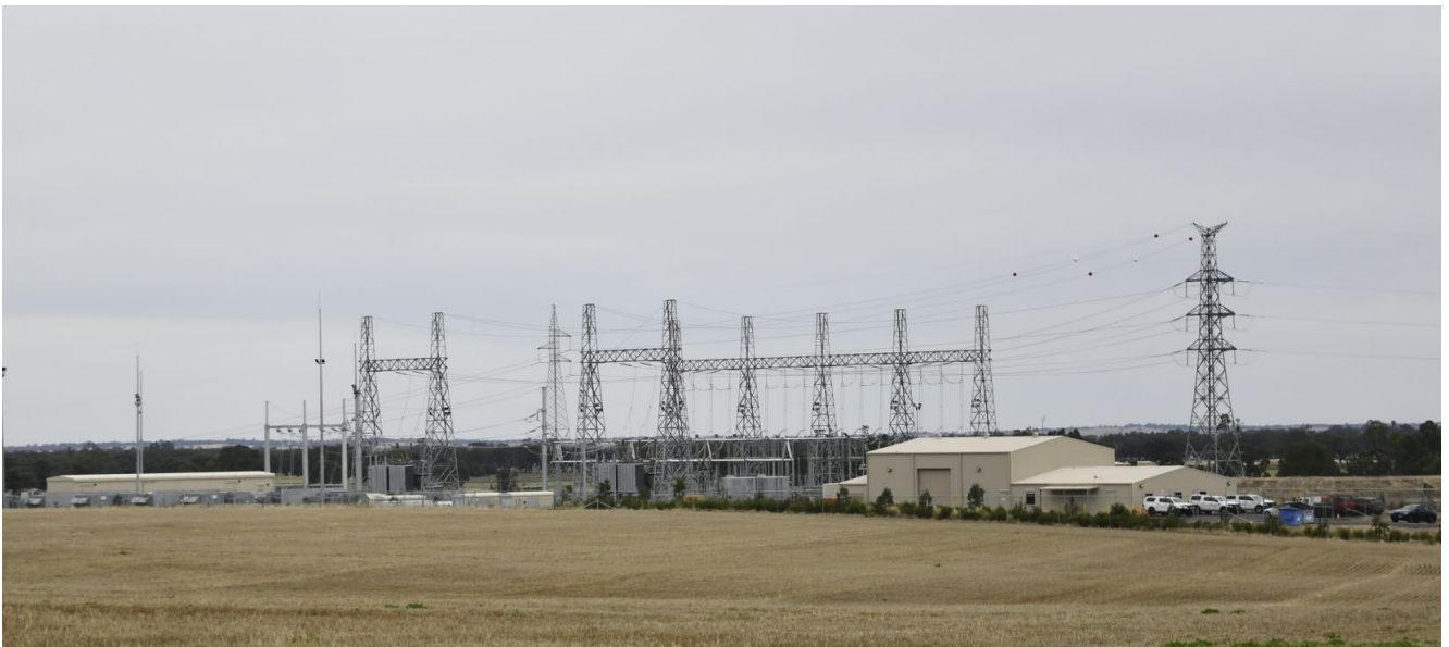
Figure 3-3: Typical terminal station
