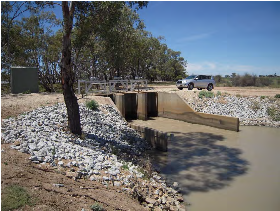
Figure 1 Third Reedy Lake outlet structure (to No 7 Channel)
