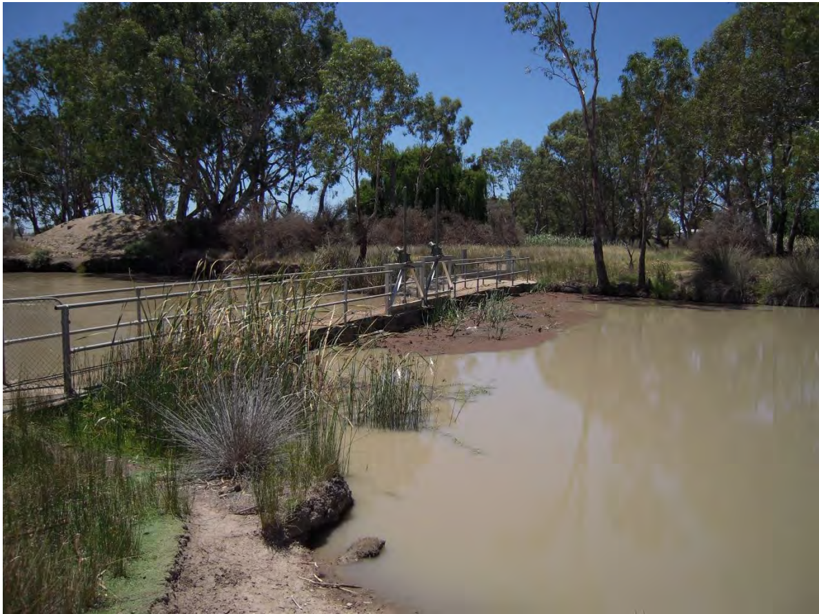
Figure 6 Regulating structure between Middle and Third Reedy Lake – to be upgraded.
