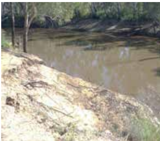
Figure 7 Left bank looking downstream of the crossing for options 2B and 2D. Exposed banks and small amounts of overhanging timber can be observed.
