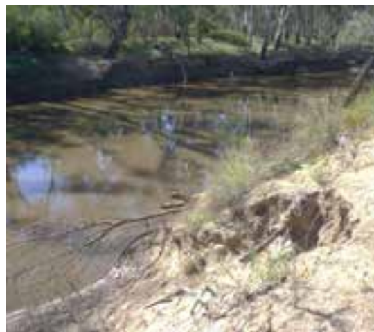
Figure 8 Left bank looking upstream of the crossing for options 2B and 2D. Exposed banks and small amounts of overhanging timber can be observed.
