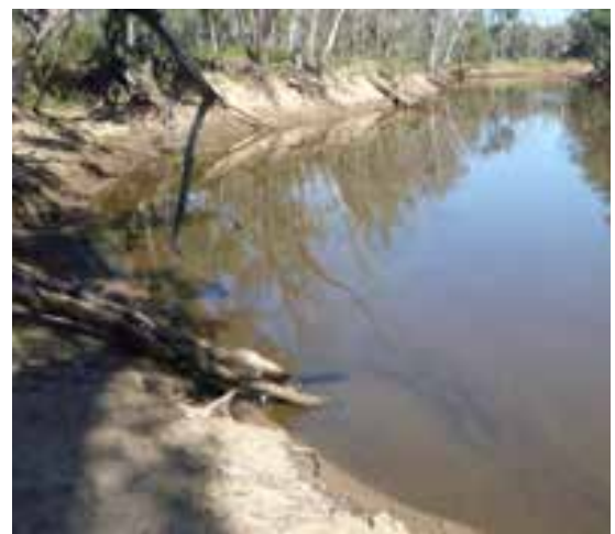
Figure 6 Left bank. Scour was observed which has potentially resulted from the instream structure observed at this location
