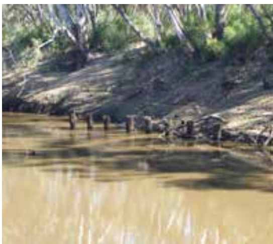
Figure 5 Pylons from old instream bridge or other structure on right bank
