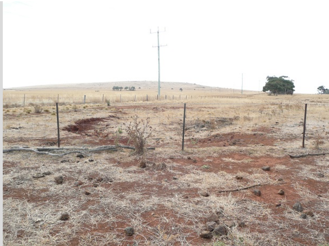
5. Facing downstream at Upstream Dam. Note active erosion along top of bank. Greens Hill located in centre background.
