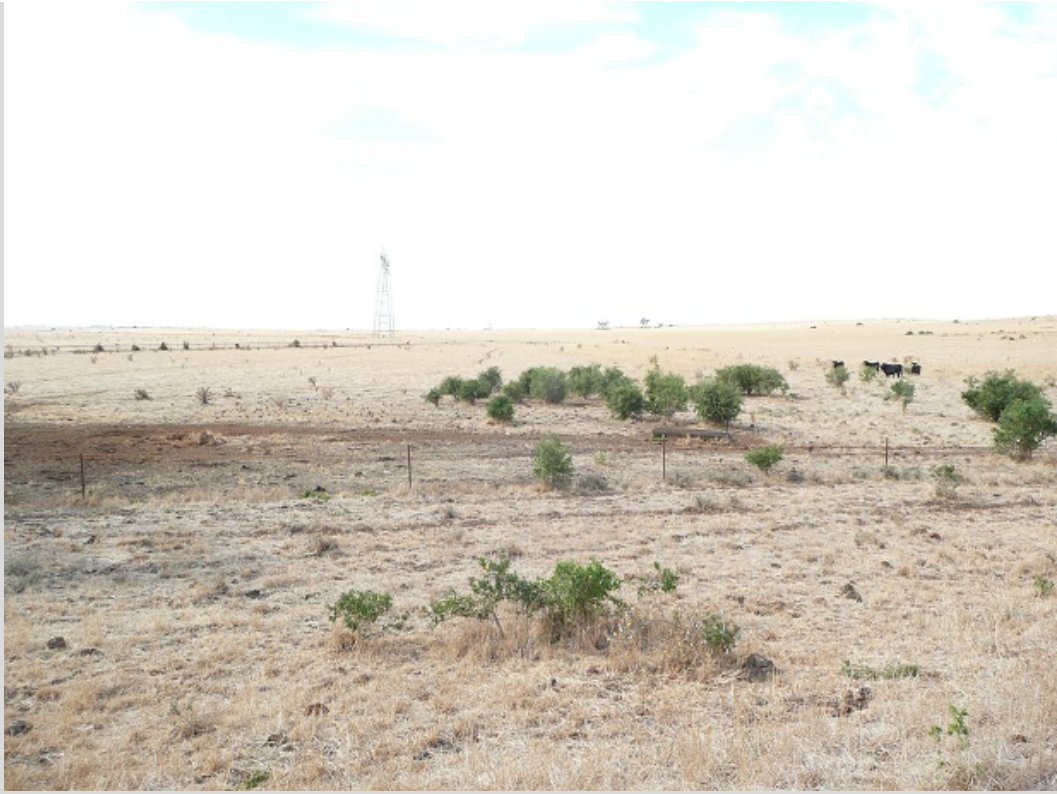
9. Facing south from the downstream side of Lower Dam. Note local depression and stock erosion. Transmission line in centre
