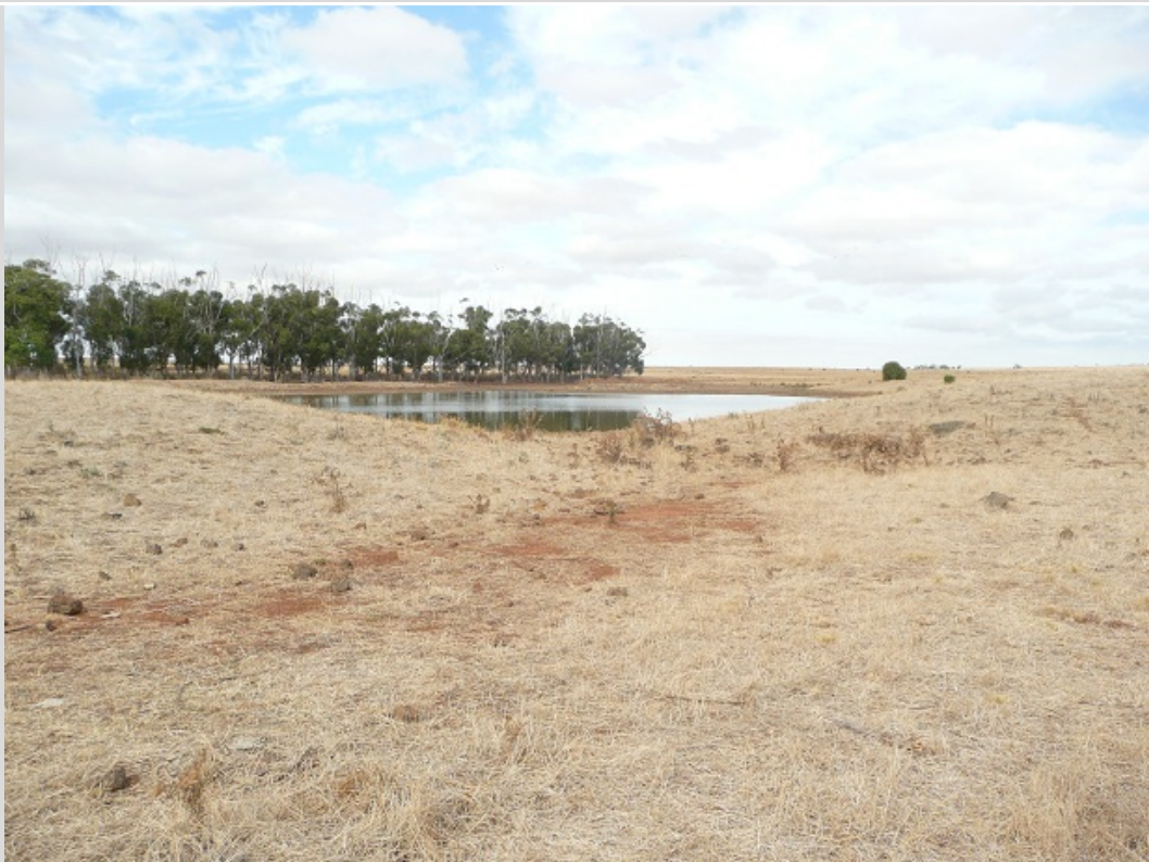
4. Upstream Dam, facing west (upstream). Dam in background and overflow in foreground.
