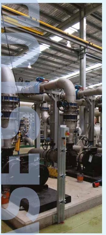
The Altona Recycled Water Project involved designing, constructing and operating an ultra-filtration and reverseosmosis plant to produce two grades of recycled water from secondary treated water produced at the Altona Treatment Plant.
