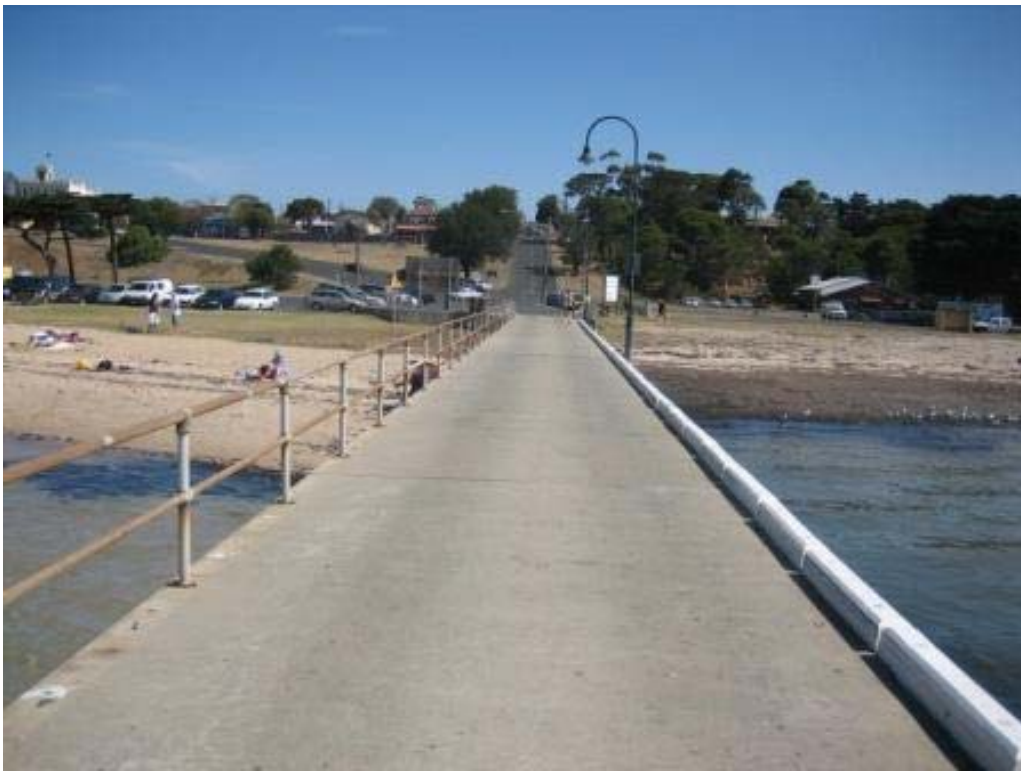
Figure 2-12 Impact of Groyne Alongside Portarlington Harbour Pier
