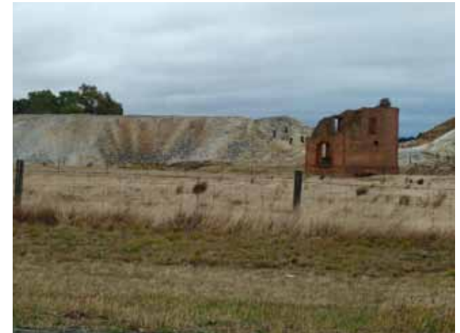
1.9 Remains of the Pumphouse
