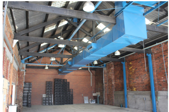
Figure 12 Interior space with later ventilation and lighting.
