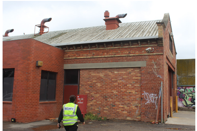
Figure 8 Detail of southern facade, note the alteration of existing openings.
