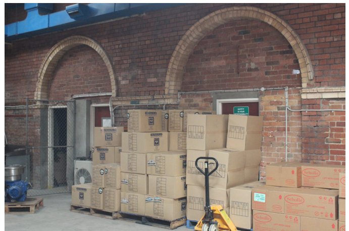
Figure 6 Internal view of the western elevation showing remnant arched opening which have been infilled.
