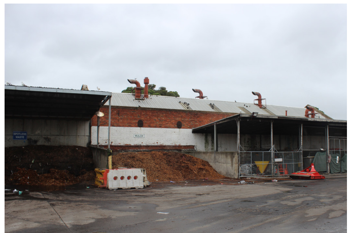
Figure 10 General view of the northern facade. Note the new open structures.
