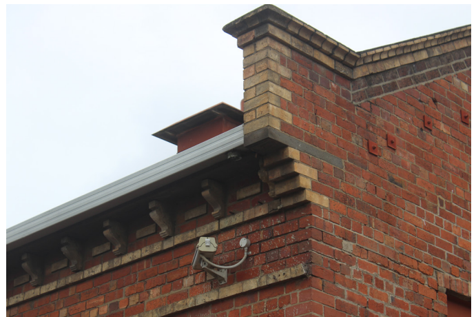
Figure 4 Detail of the eastern gable end. Note the decorative brick detailing on both the east and southern elevations.
