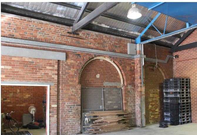
Figure 9 Detail of the remnant arched openings on the southern facade.
