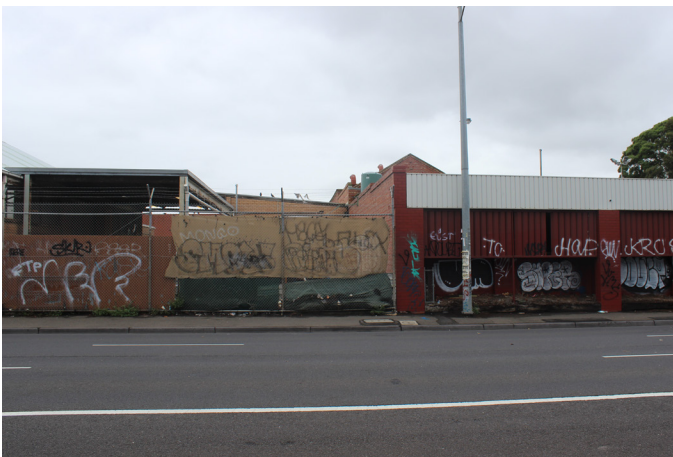
Figure 5 View of the western gable end and 1960s buildings from George Street.
