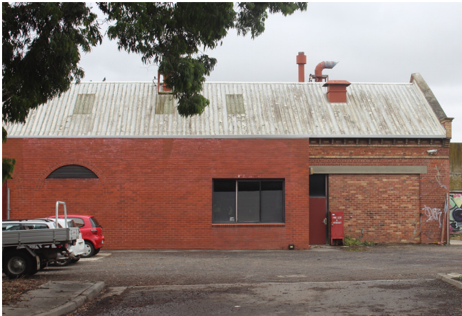
Figure 7 South facade, showing 1960s building abutting the Gas Store.
