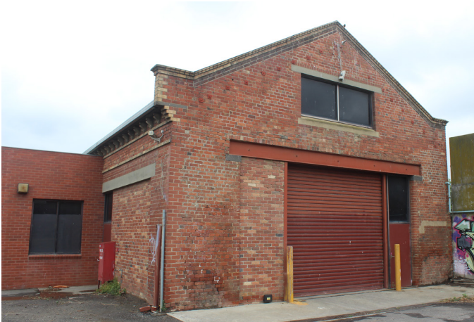
Figure 3 View of the eastern gable end from within the site. Note the extensive alterations creating the current roller door arrangement.
