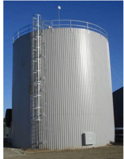
Heat Buffer Tank
