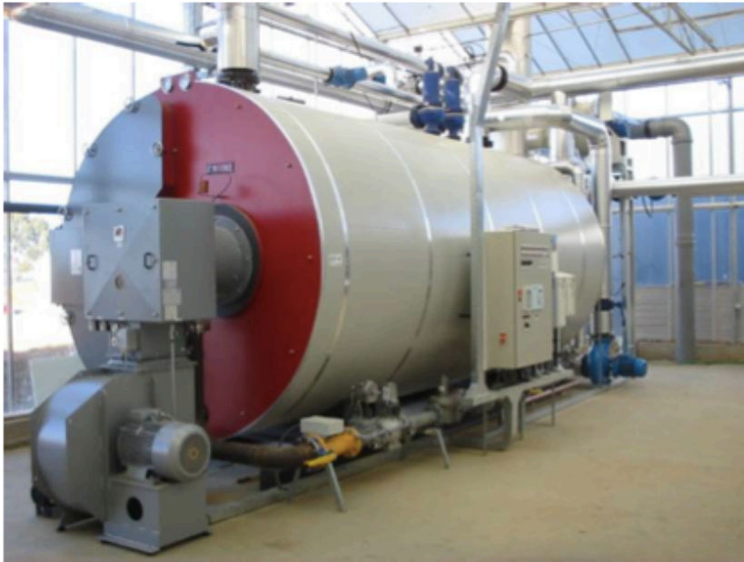
Natural Gas Boiler System
