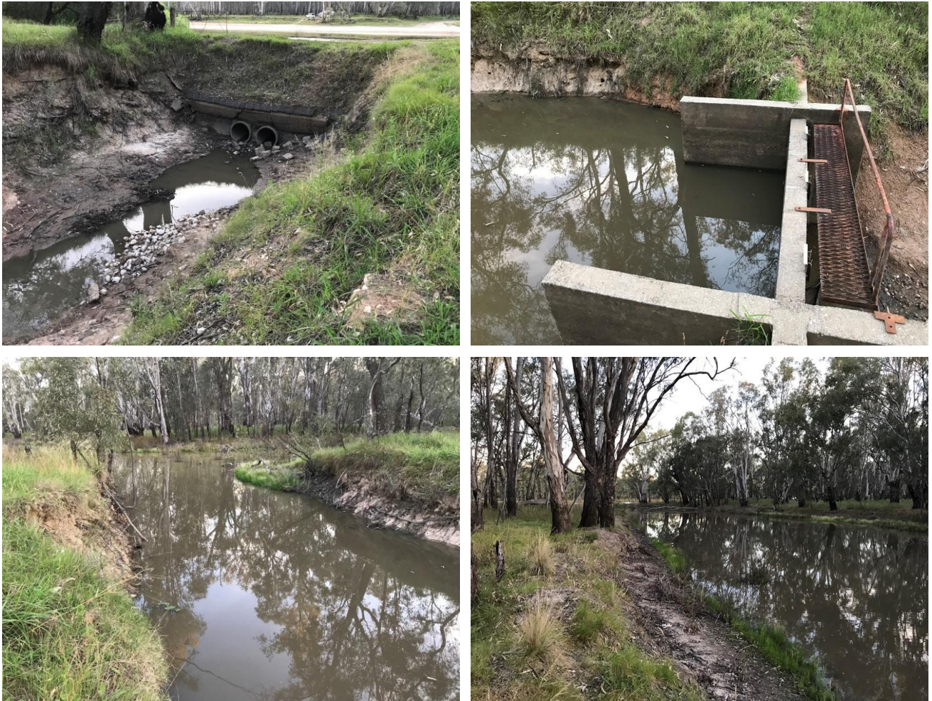
Figure 2-5 The existing regulator and pump station. Top left: pipe through embankment, looking towards the Murray River. Top right: Regulator structure controlling water level in Lake Moodemere. Bottom left: Arm of Lake Moodemere facing east, away from the Murray River. Bottom right: Lake Moodemere, near the regulator.
