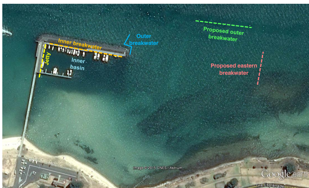
Figure 7. Locations inspected by CEE
