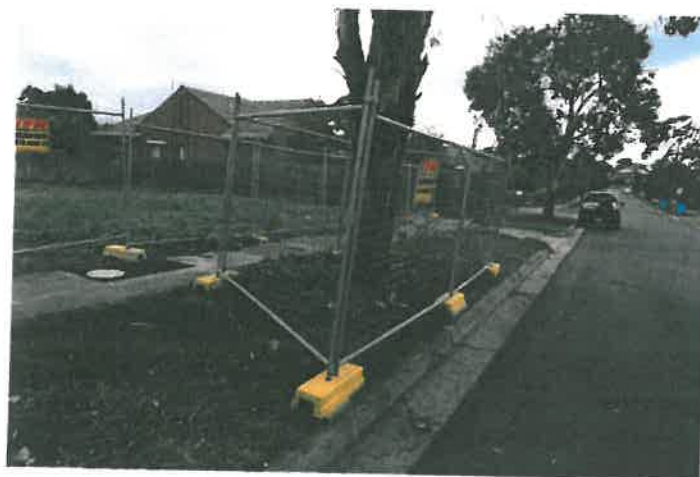
Photograph above left - Example of signage for TPZ. Photograph above right - Example of appropriate TPZ fencing.
