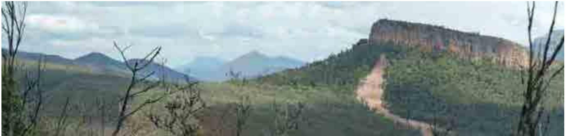
Landslip on the Mount William Range occurred after heavy flooding
