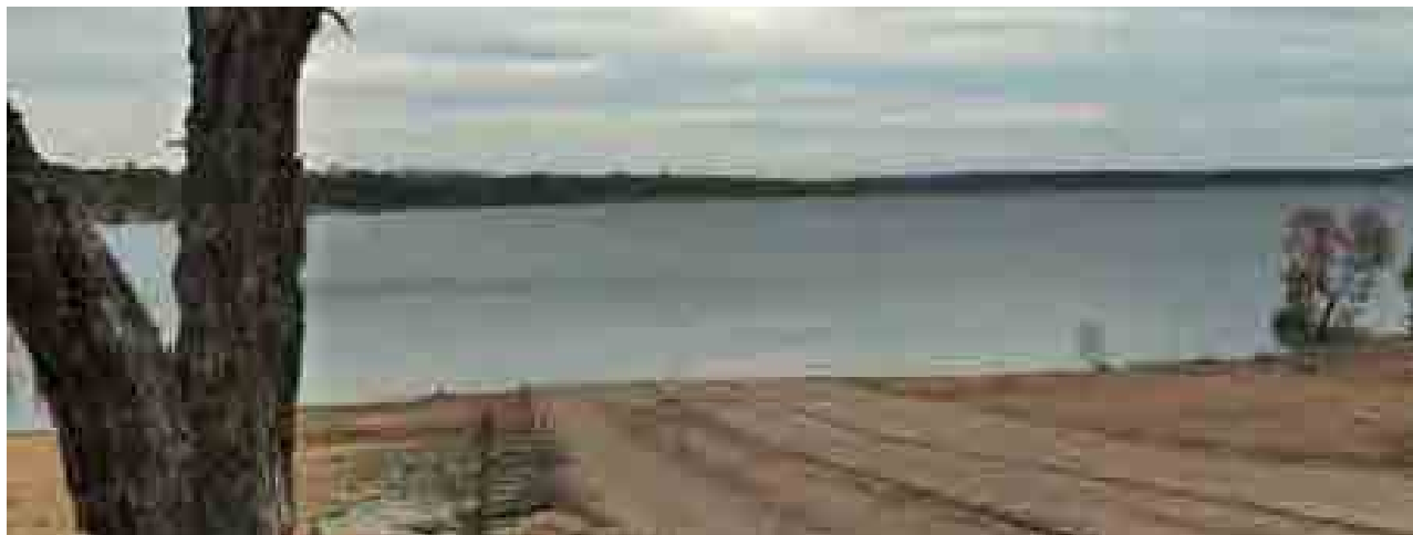
Rocklands Reservoir was created by damming the Glenelg River as part of the Wimmera Mallee Stock & Domestic Water Supply
