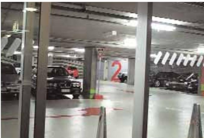
PROVIDE CLEAR, SAFE PEDESTRIAN PATHS IN CAR PARKING AREAS. USE LIGHT COLOURED PAINT AND CEILING LIGHTS TO MAXIMISE LIGHT DISTRIBUTION.
