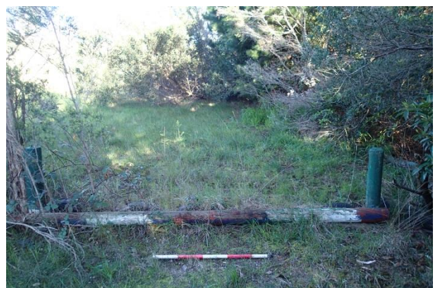
Plate 26: Pony Club infrastructure located adjacent to northern boundary, facing west
